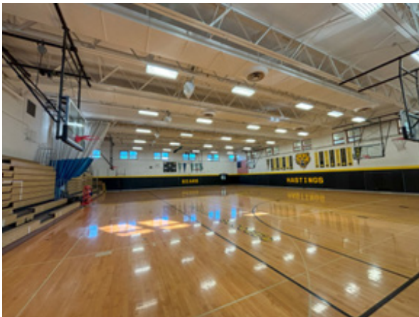
Gymnasium in need of air conditioning
