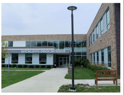
Wickliffe Elementary School Rebuild
