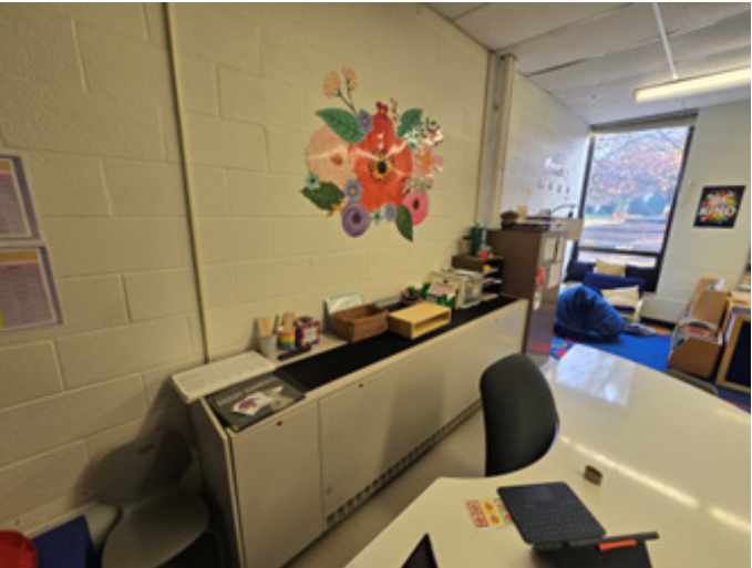
Classroom unit ventilators are original to the building, noisy, disruptive to teaching and inefficient.
