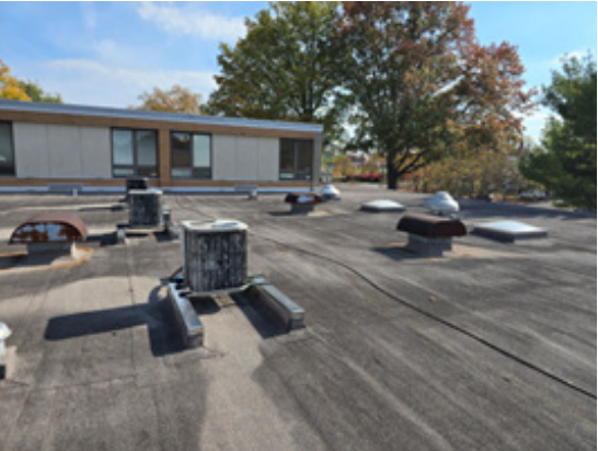
Roof replacement required with proper slope for water drainage
