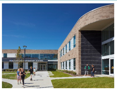
Windermere Elementary School Rebuild
