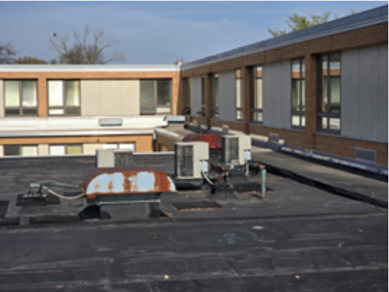
Roof replacement required with proper slope for water drainage
