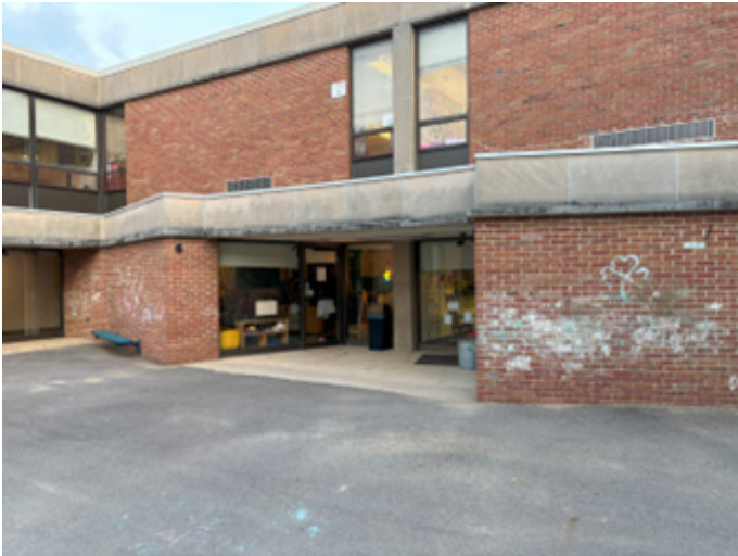
Original non-insulated single pane aluminum windows with limited daylighting in each classroom.
