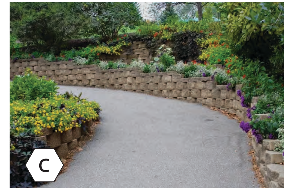
Segmental retaining wall
