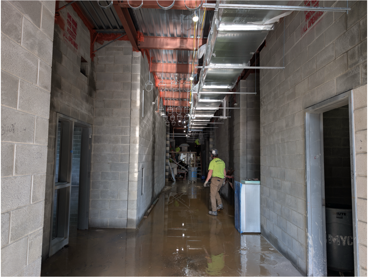
Progress in the North Wing
