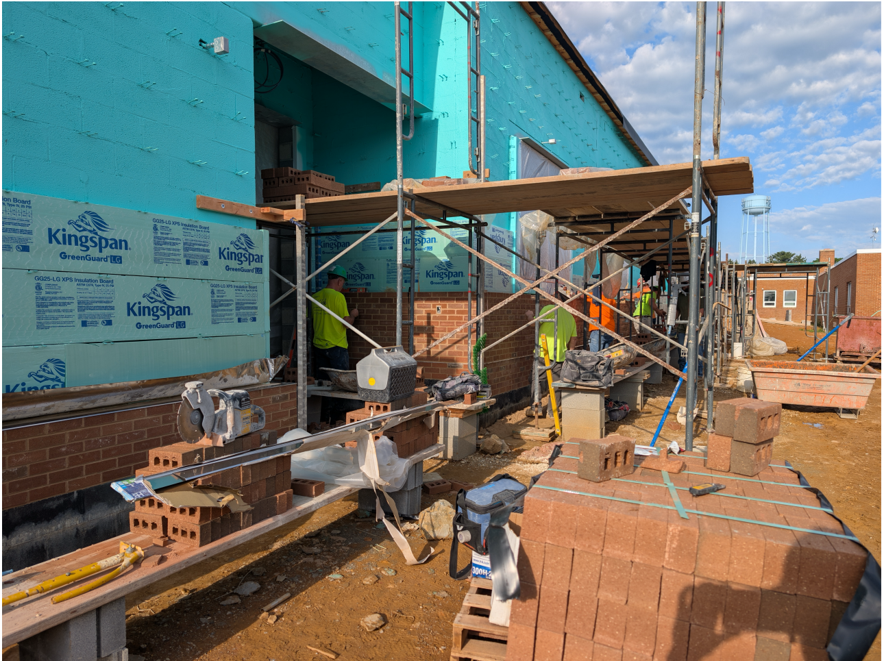
Brick Progress Courtyard of New Addition
