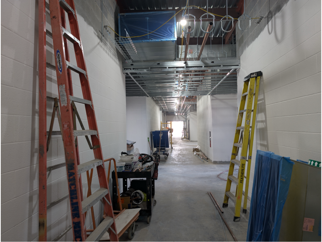
South Wing Progress
