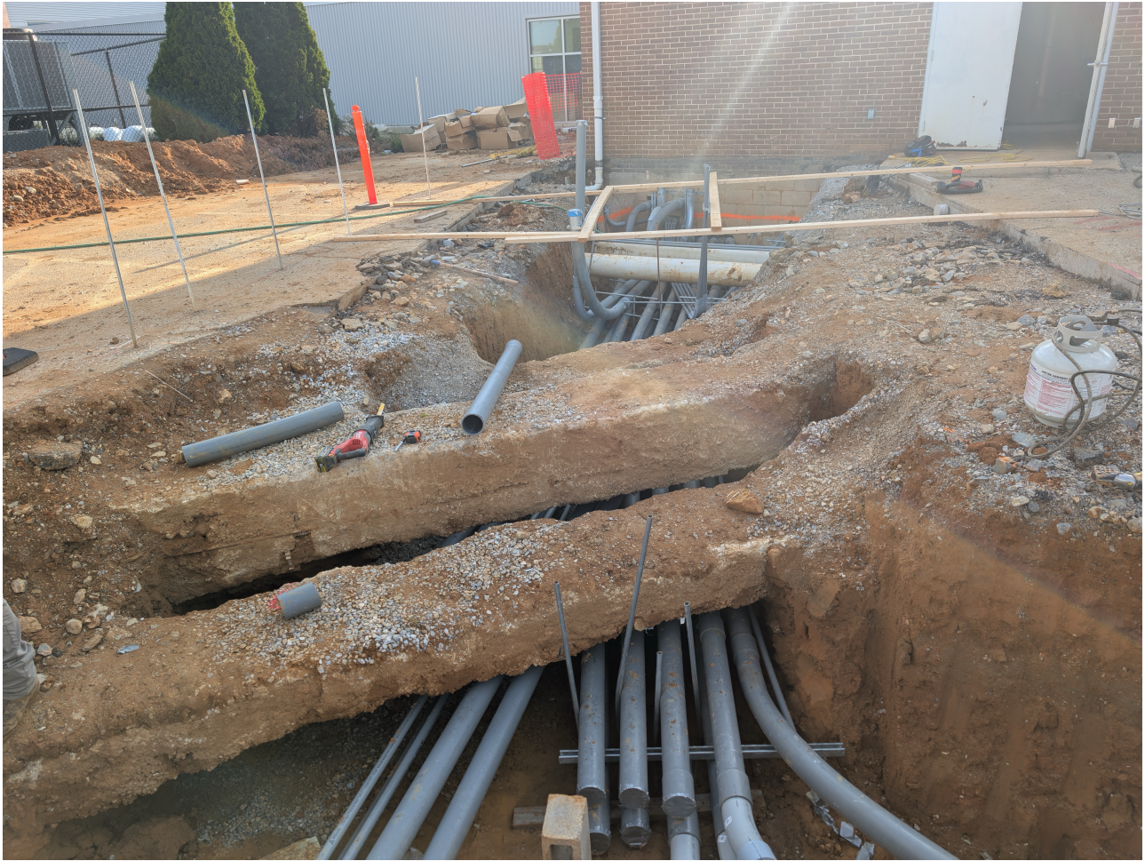
New Electric Conduit Runs into New Electric Room
