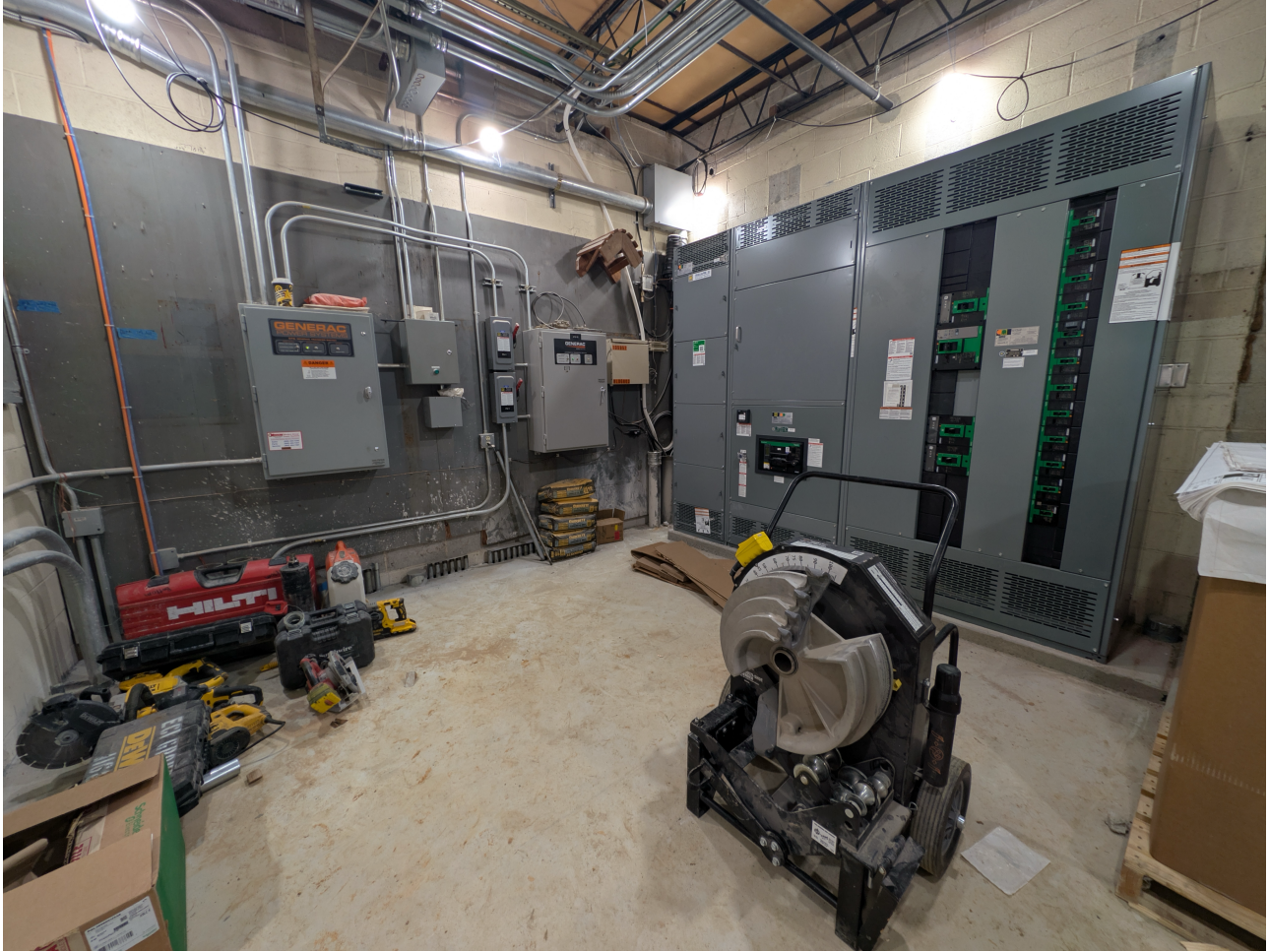
New Electric Room Equipment Set in Place
