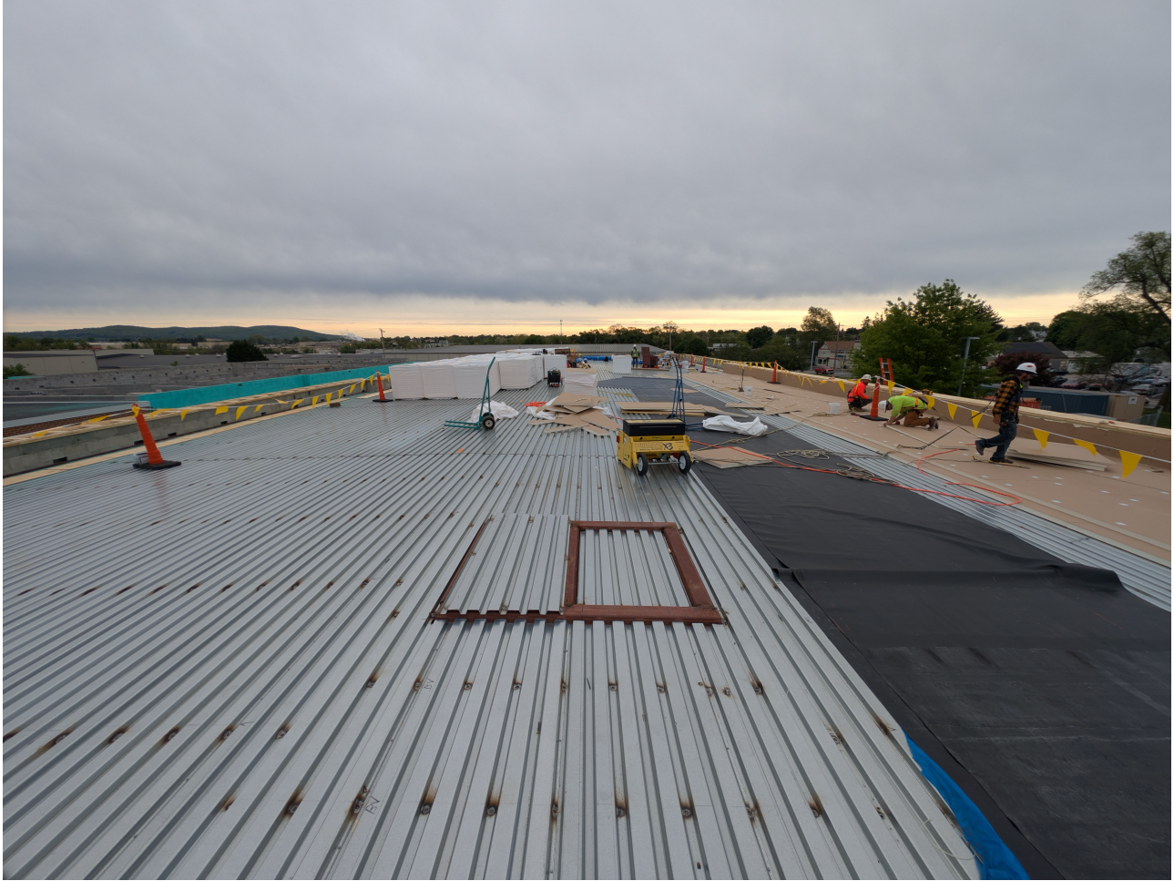
Roof Progress South Wing Area D Addition
