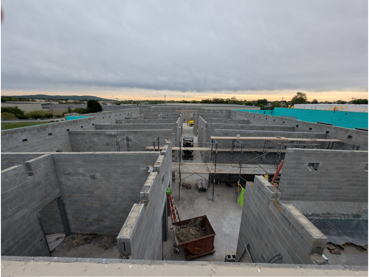
North Wing Area D Addition Progress
