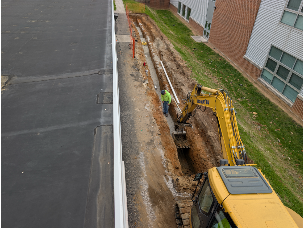
Sewer Line Excavation Behind 2 nd Grade Wing
