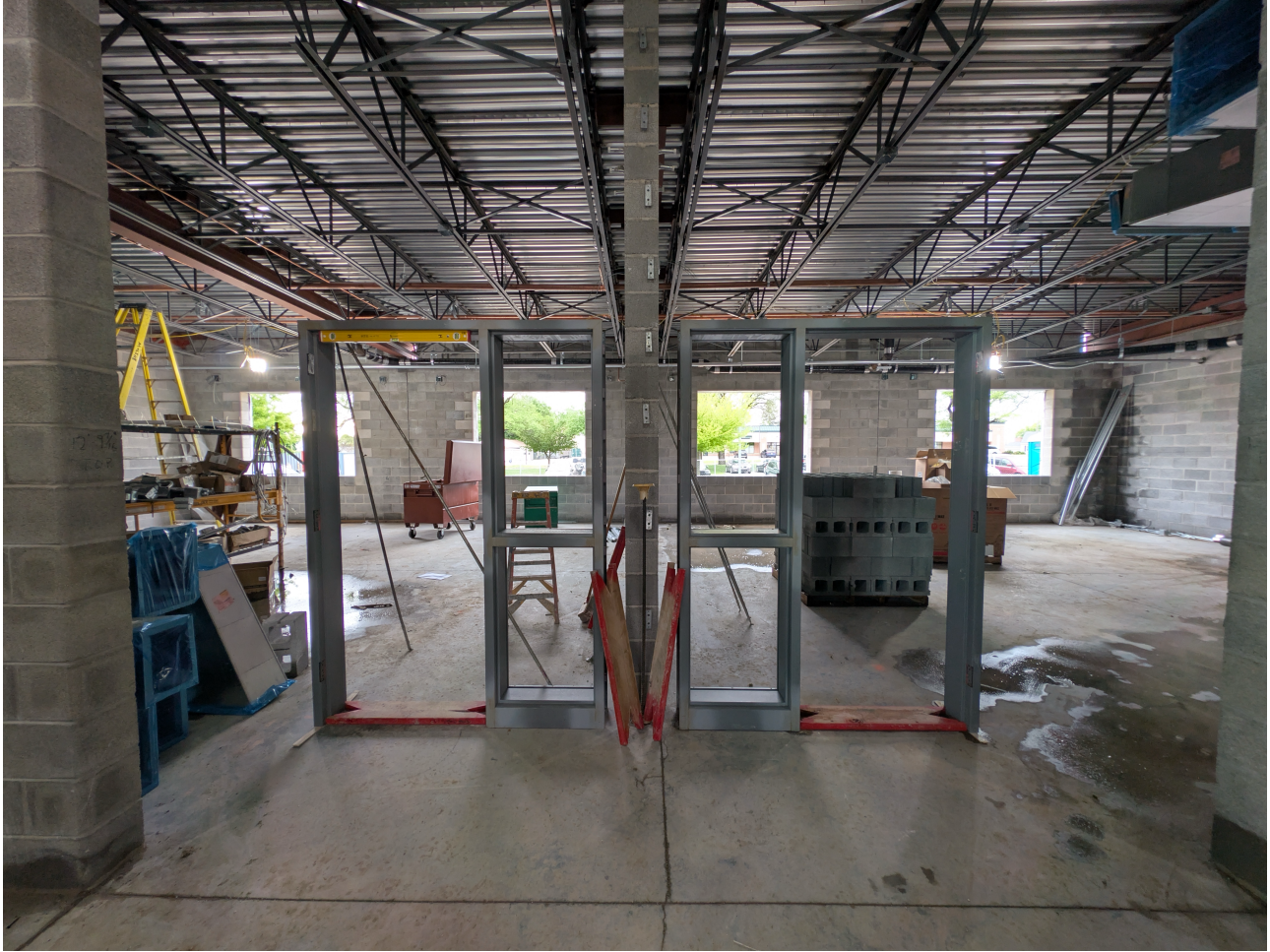
Classroom Entryways South Wing Area D Addition
