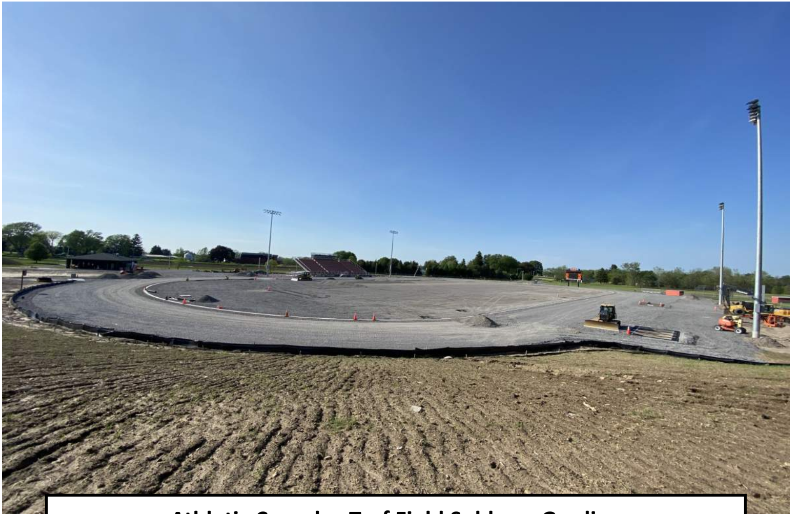
Athletic Complex Turf Field Subbase Grading
