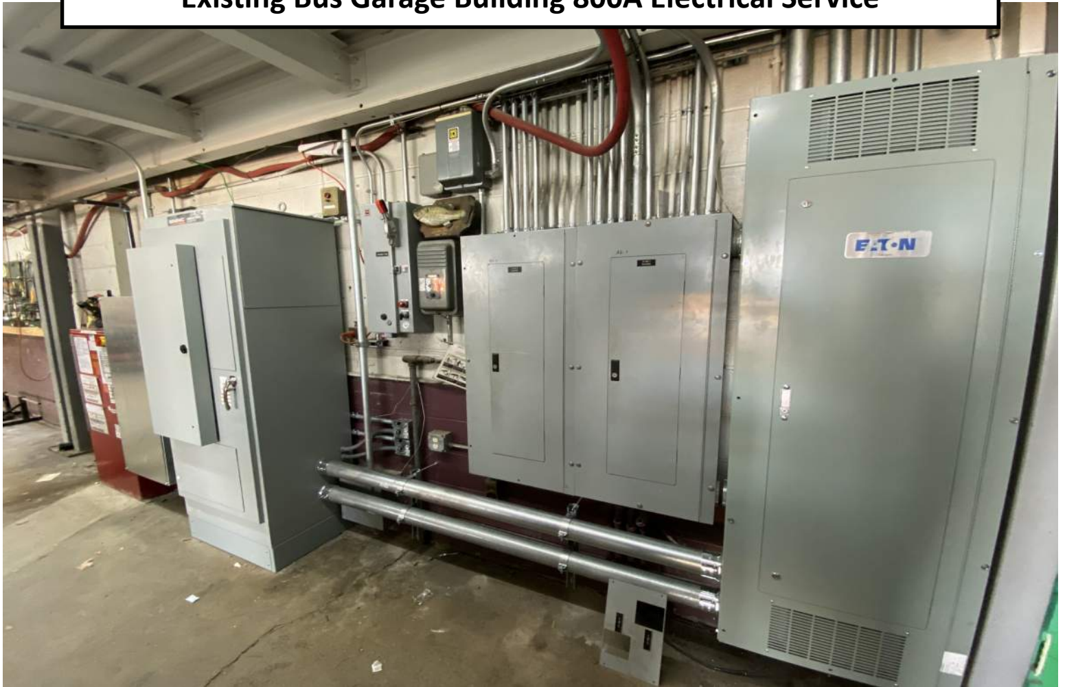
Existing Bus Garage Building 800A Electrical Service
