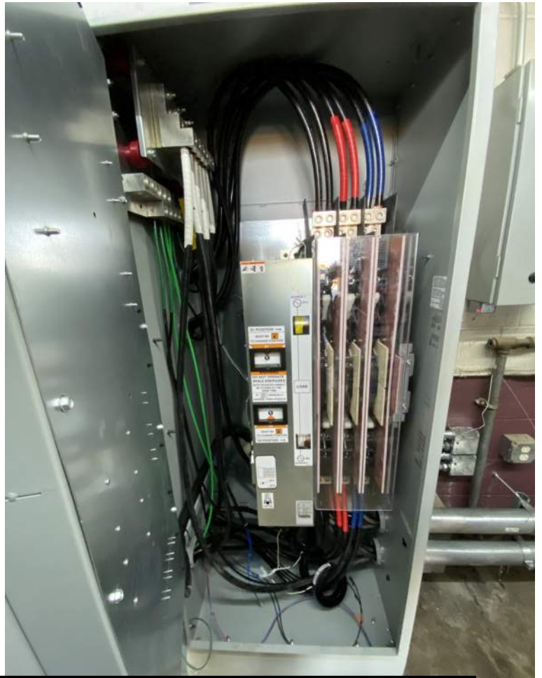
Existing Bus Garage Building 800A Electrical Service
