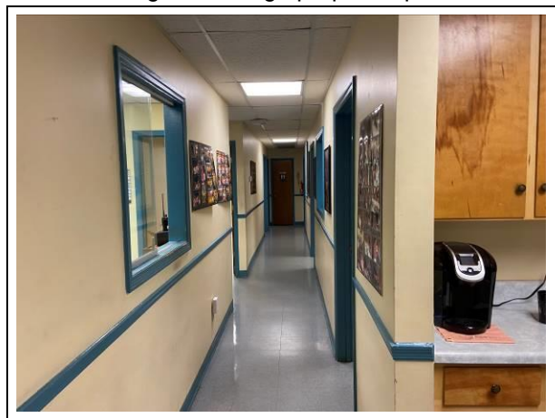
Photo #12. View of typical assumed ACBM materials in the hallway of the office.
