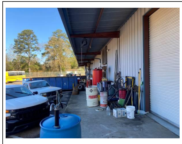
Photo #16. View of typical metal exterior siding observed around the building.
