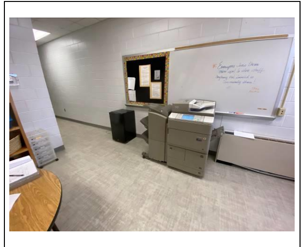
Photo #8. Typical non-detect light/dark gray LVT flooring in 200 hall teacher work room.
