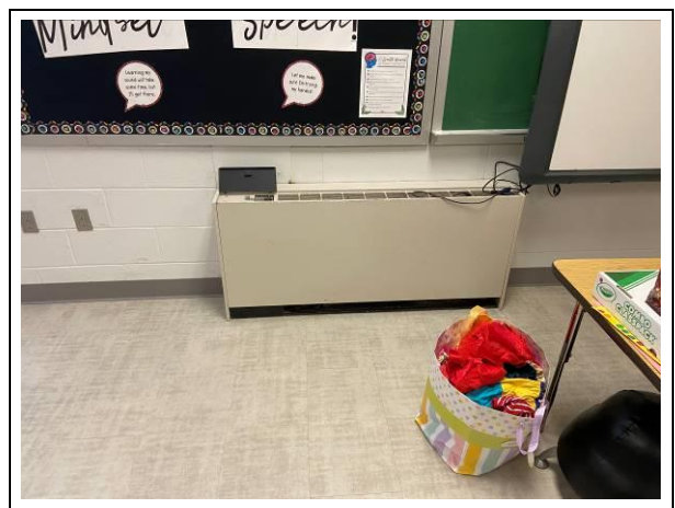
Photo #6. View of non-detected gray cove base with yellow mastic and light/dark gray LVT with yellow mastic sampled during February 2022 inspection.
