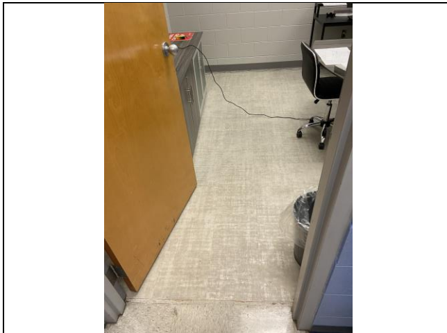
Photo #3. View of typical non-detect light/dark gray luxury vinyl flooring (LVT) in office conference room.
