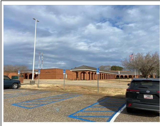
Photo #1. Northwest view of typical exterior building Materials observed along main entrance to school.
