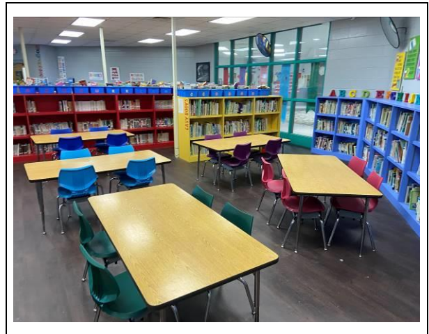
Photo #10. Another view of typical interior finishes observed in the media center.
