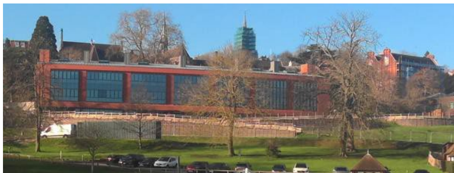
Fig 1: Harrow's bespoke new Biology and Chemistry building
