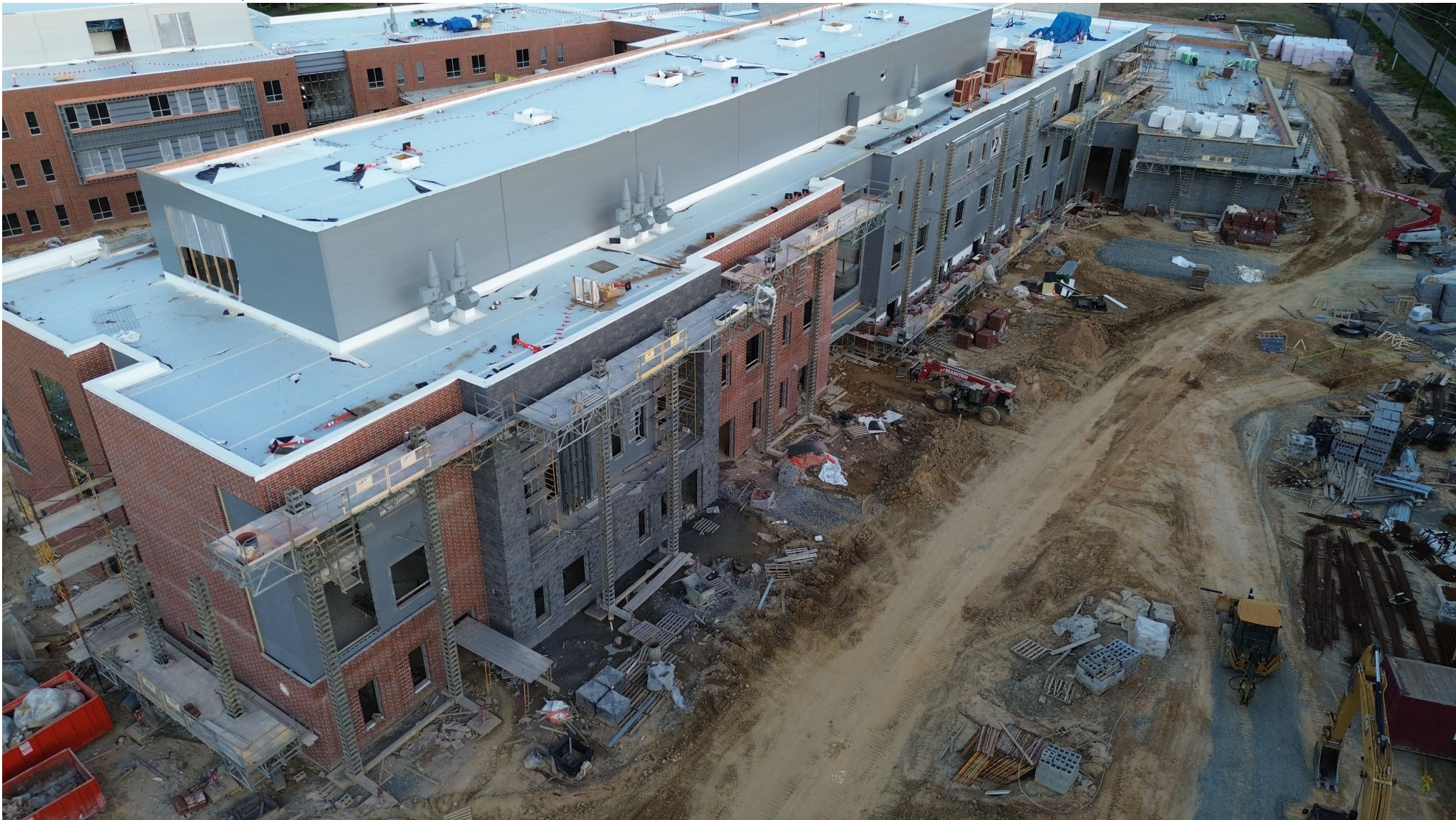
NORTH EAST MIDDLE / HIGH SCHOOL – REPLACEMENT – HIGH SCHOOL WING – EXTERIOR BRICK AND STONE INSTALLATION
