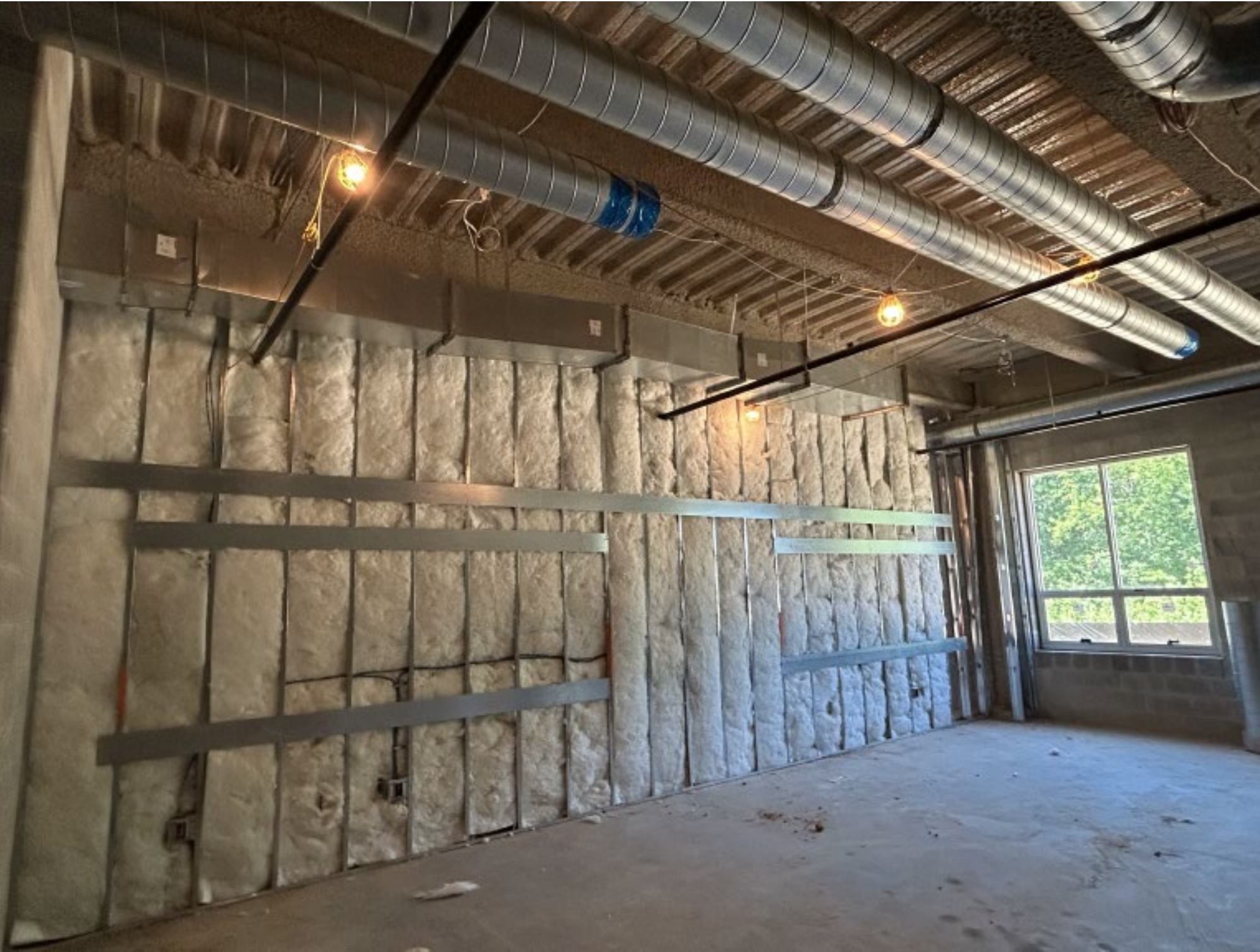
NORTH EAST MIDDLE / HIGH SCHOOL – REPLACEMENT – AREA C – MIDDLE SCHOOL WING – WALL INSULATION
