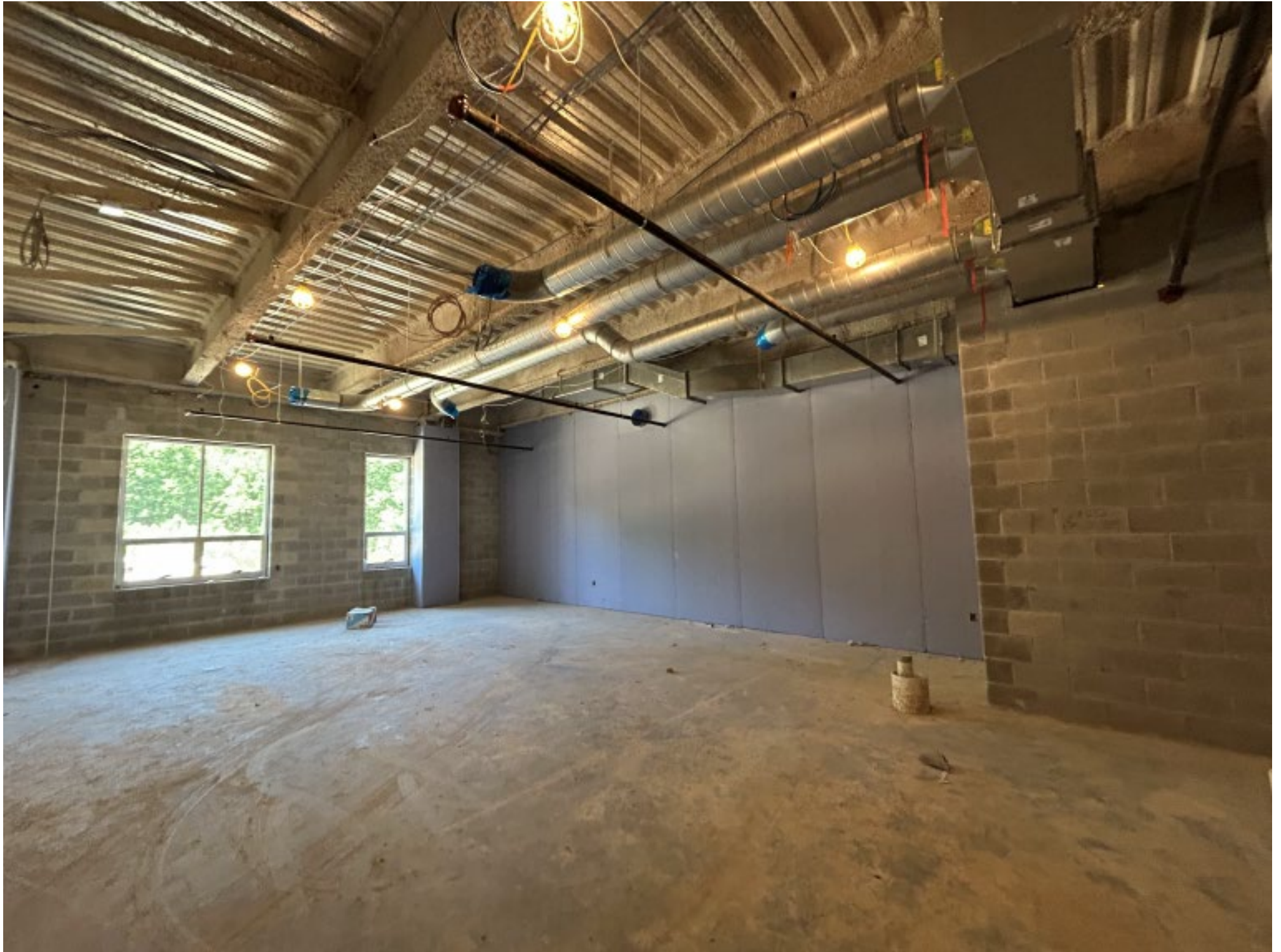
NORTH EAST MIDDLE / HIGH SCHOOL – REPLACEMENT – AREA C – MIDDLE SCHOOL WING – DRY WALL INSTALLATION
