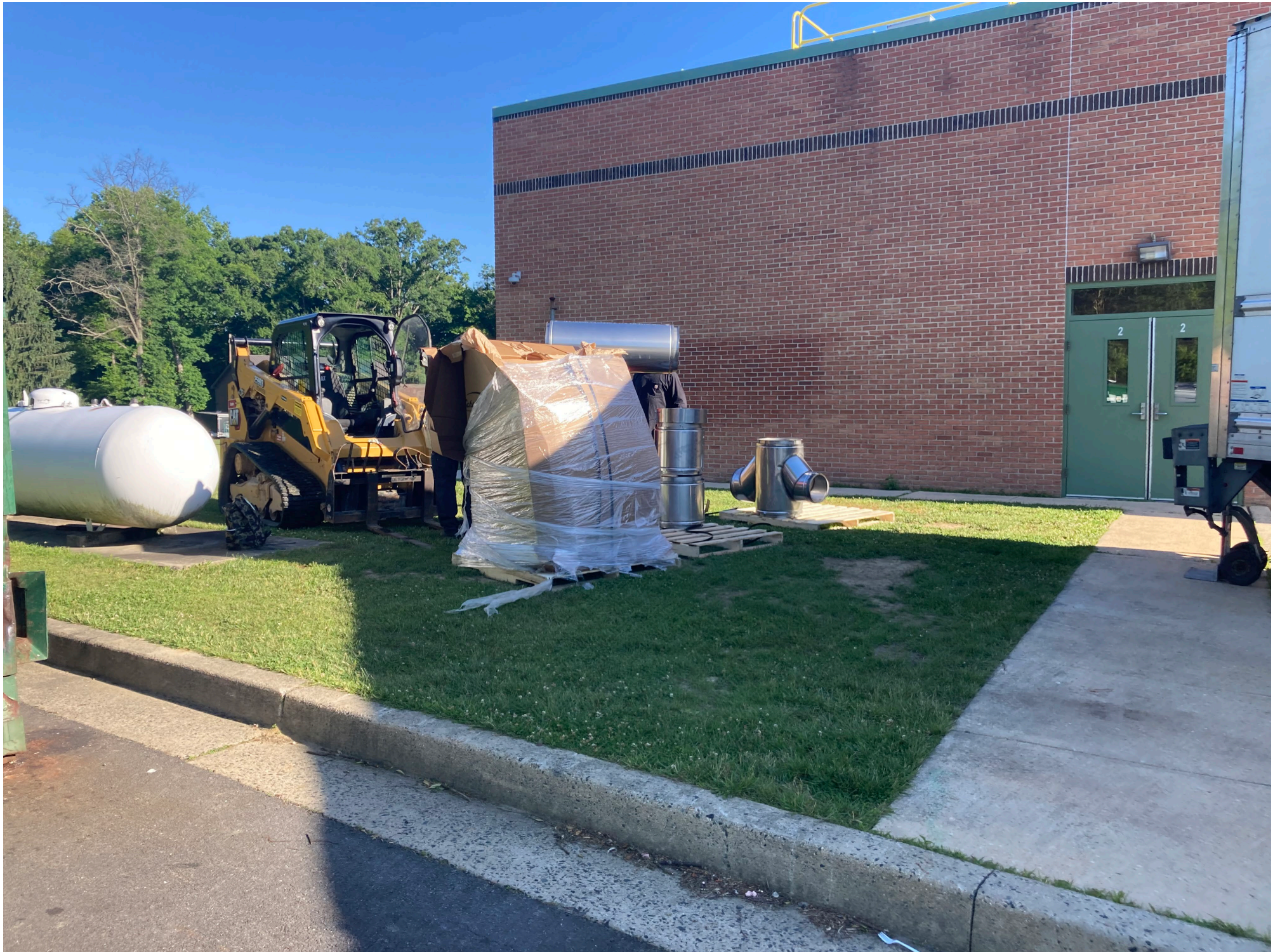
CECIL MANOR ELEMENTARY SCHOOL – HVAC REPLACEMENT
