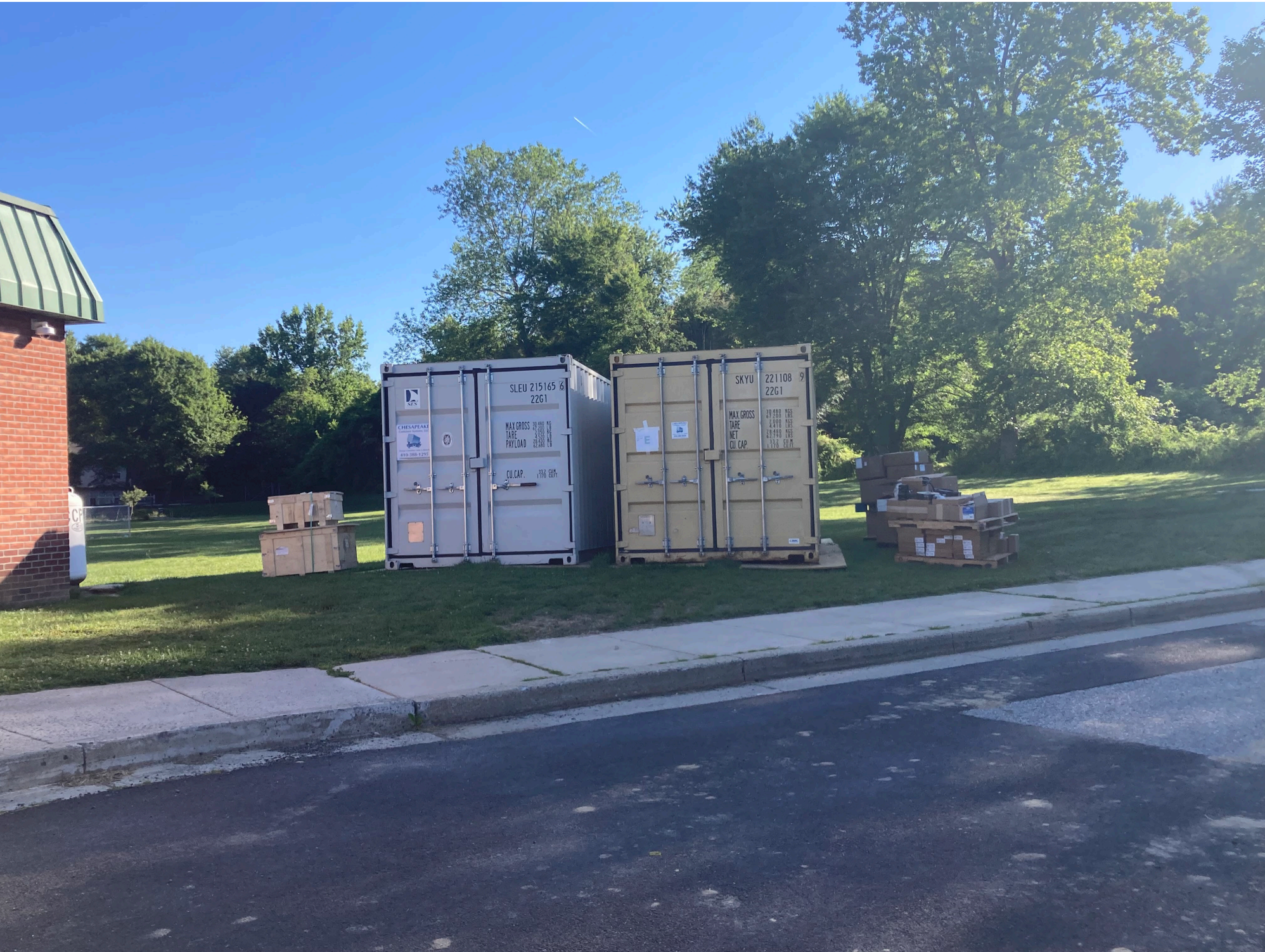
CECIL MANOR ELEMENTARY SCHOOL – HVAC REPLACEMENT
