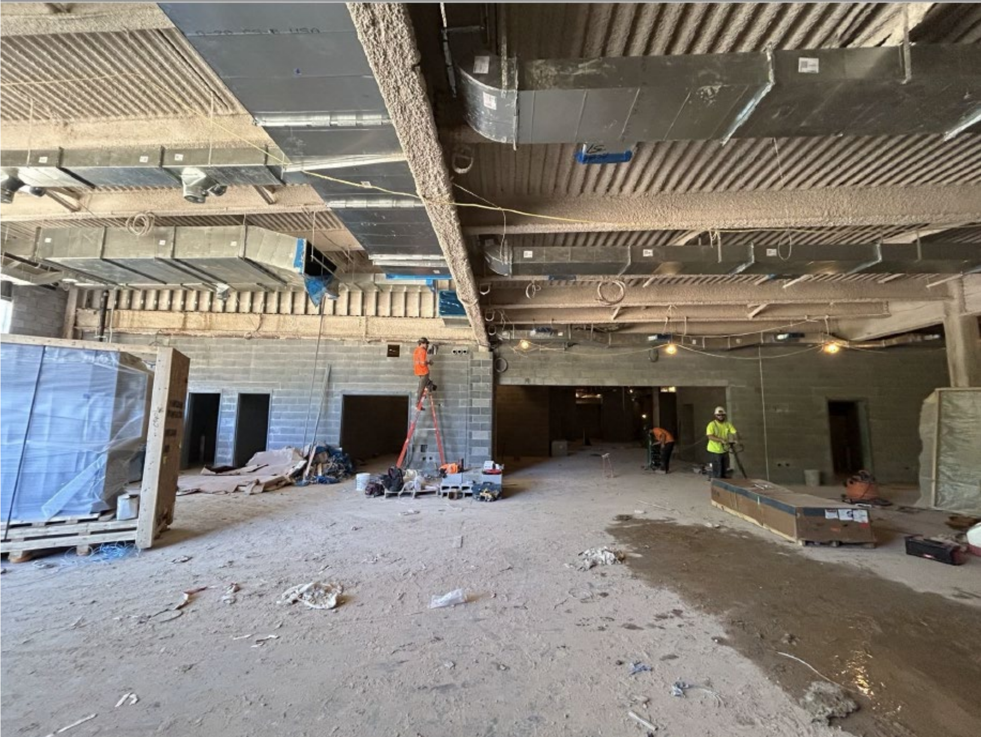
NORTH EAST MIDDLE / HIGH SCHOOL – REPLACEMENT – AREA B – MIDDLE SCHOOL CAFETERIA
