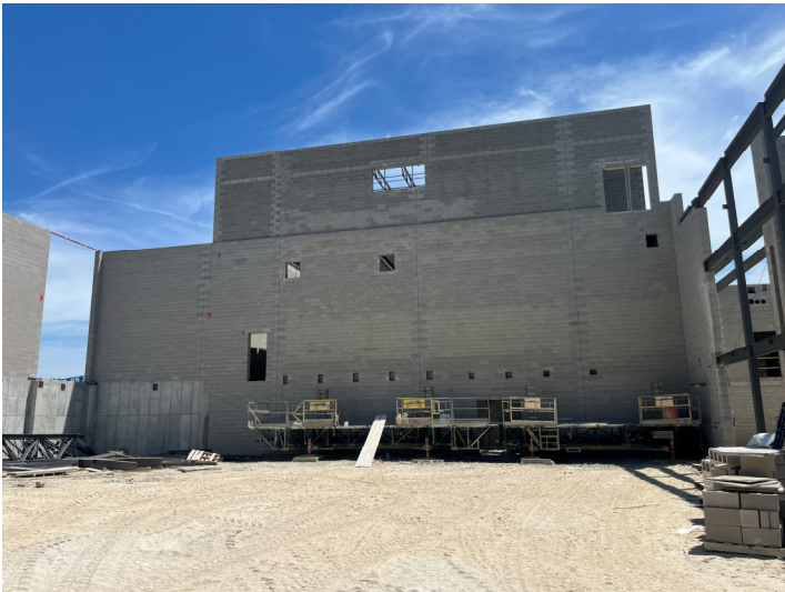
CMU Wall – East Side Of Area C2
