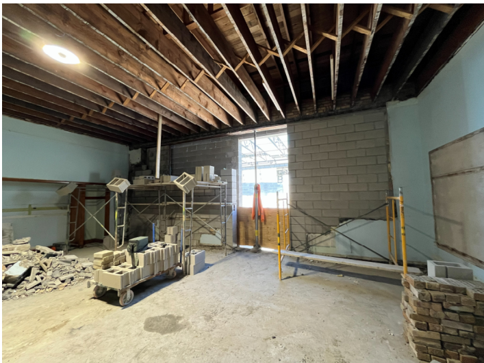
CMU Wall – Area A1
