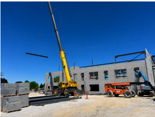
Crane Lifting Structural Steel Into Area C1
