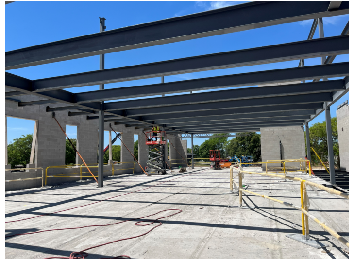
Structural Steel Installed – Area C1
