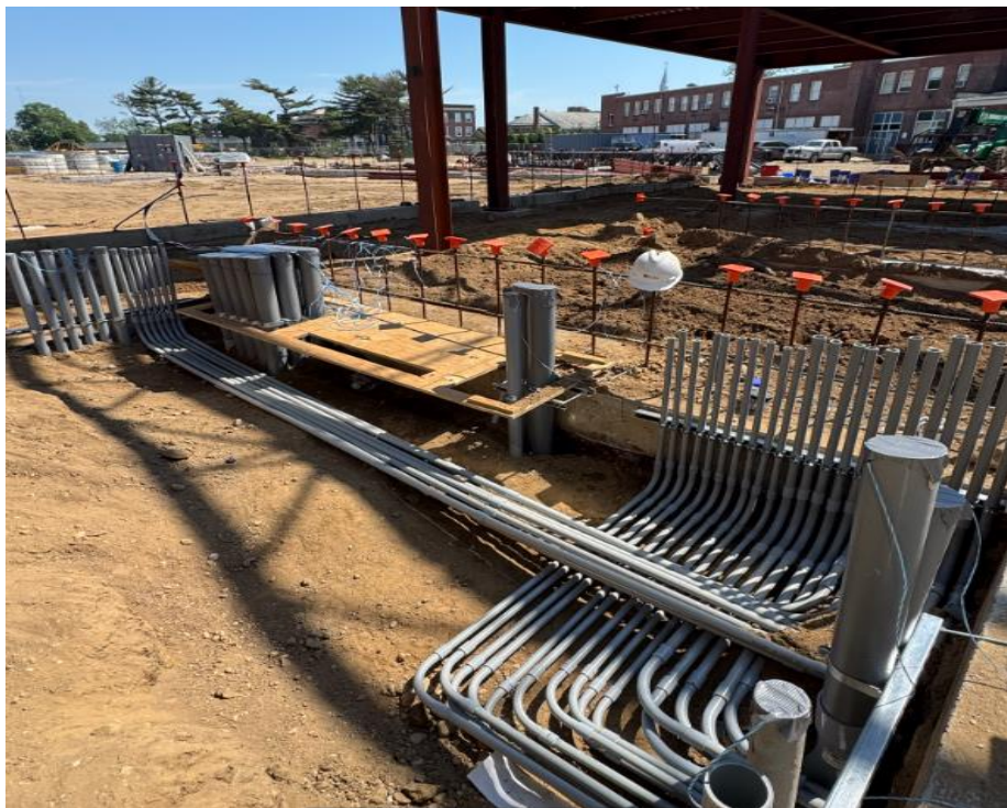
Hempstead ABGS MS – Underground Electric Roughing
