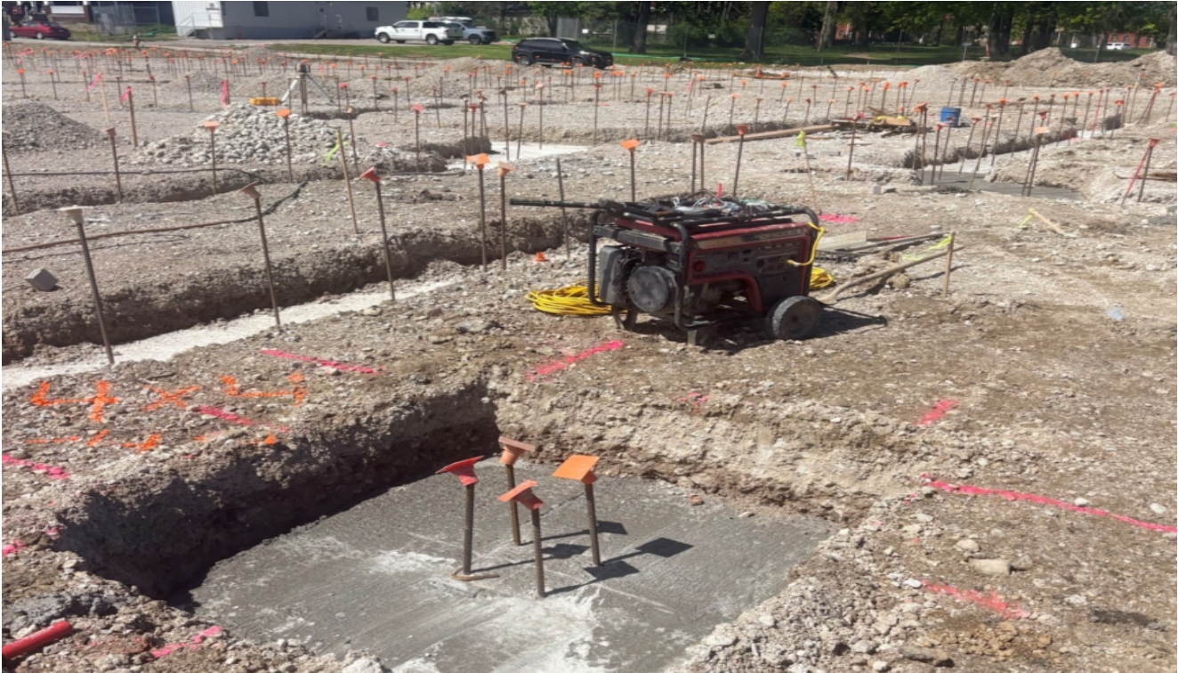
Area A, Concrete Column Pad
