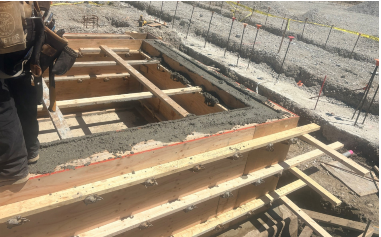
Area A, Elevator Pit wall forms and concrete placement
