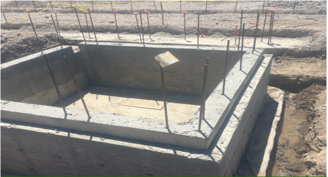
Area A, Elevator Pit Walls
