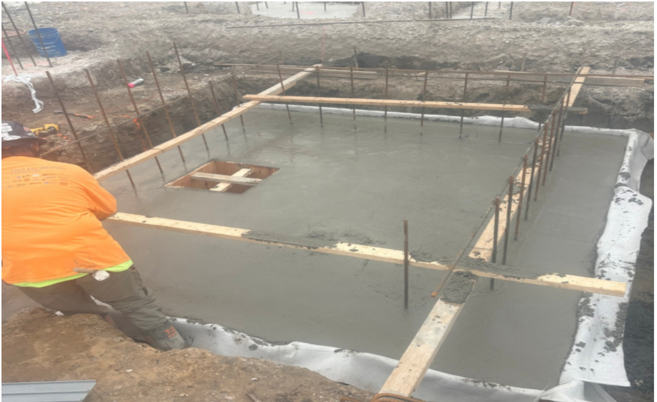
Area A, Elevator pit slab concrete placement
