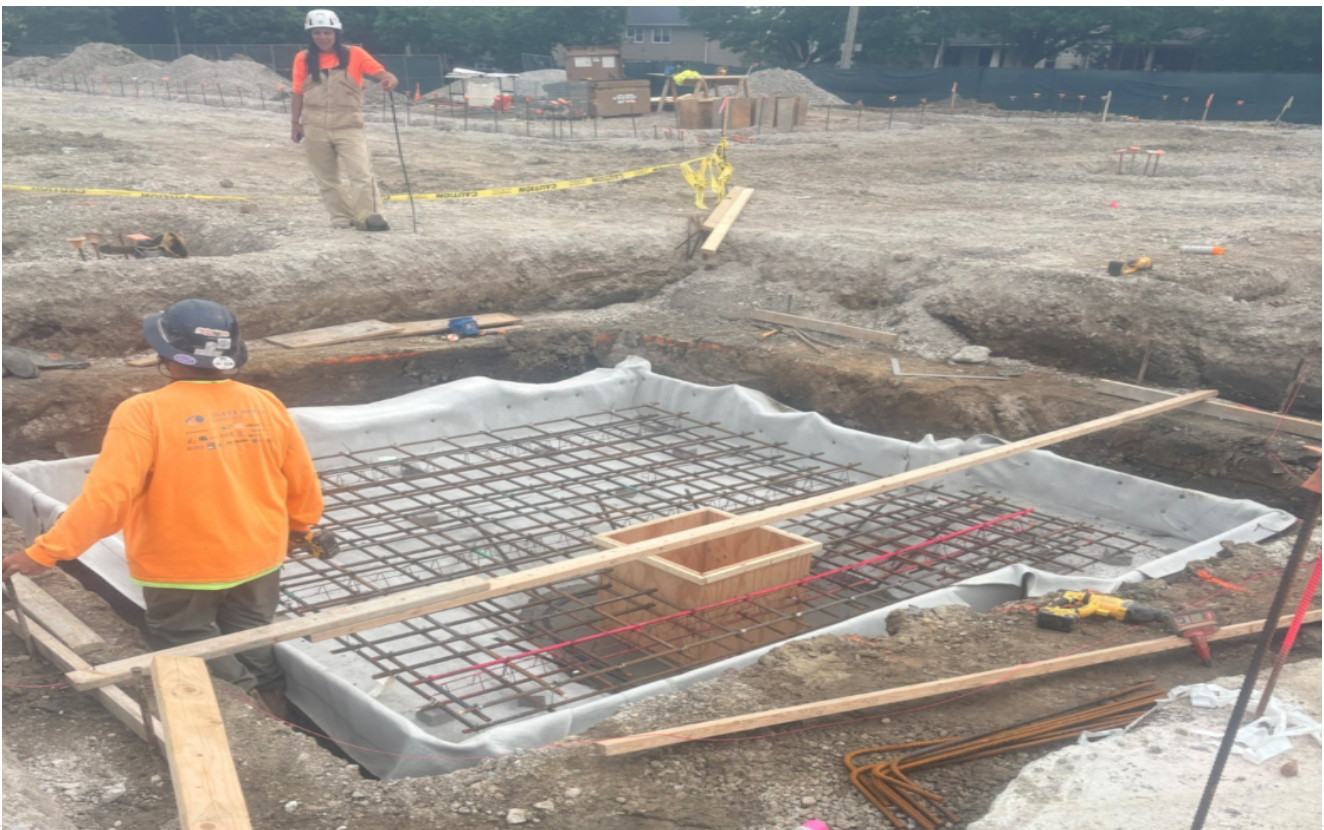
Area A, Preparation of Elevator Pit Slab
