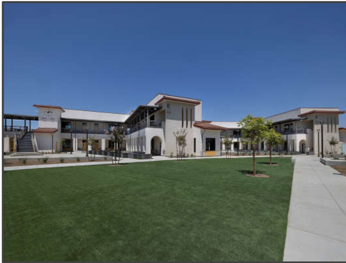
Building A & F – 2 Story Classroom
