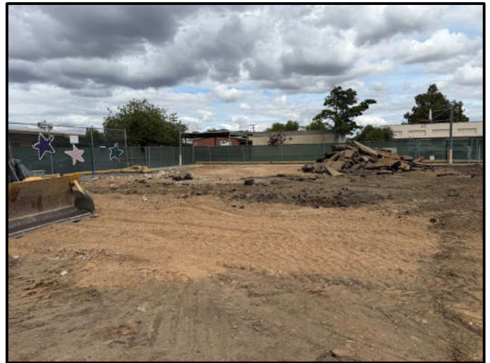
Increment 3 - Lincoln High School Asphalt Demolition
