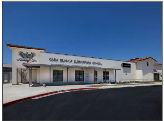
Building A - Administration Building
