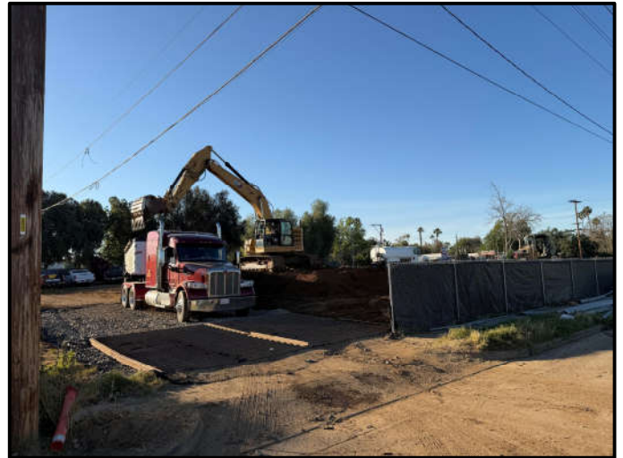
Increment 1 – Soil Mitigation Truck Loading Work
