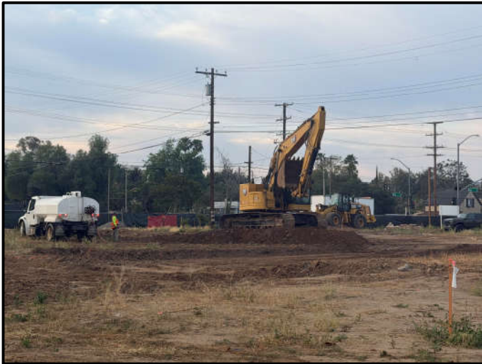
Increment 1 – Soil Mitigation Parcel C Stockpiling
