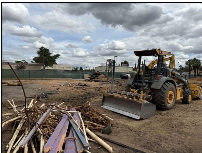
Increment 3 – Lincoln High School Demo & Site Clearing Work
