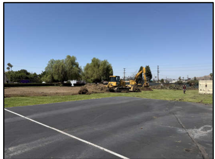
Increment 3 – Lincoln High School Grass Removal Work
