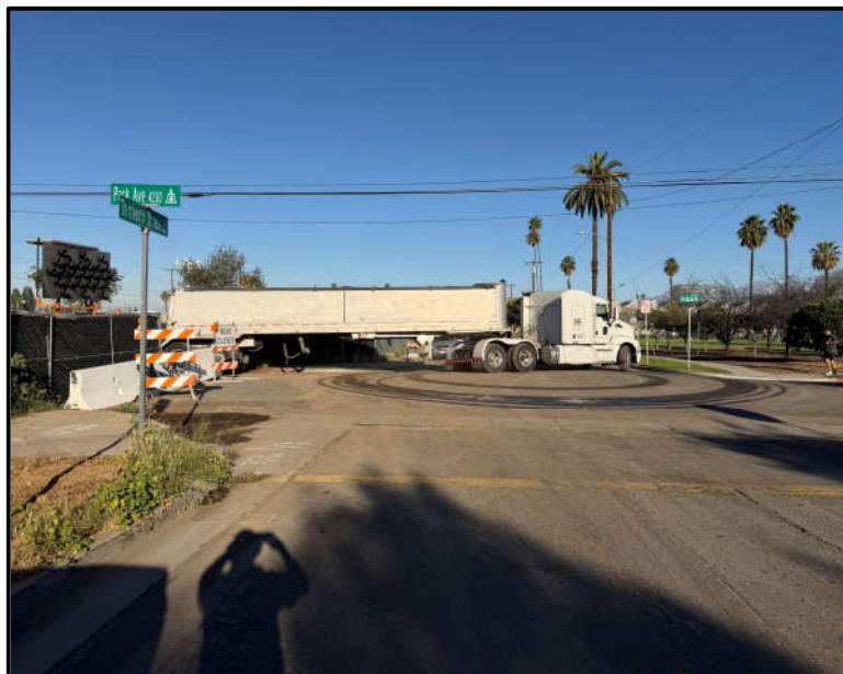
Increment 1 – Soil Mitigation Work Truck Haul Off
