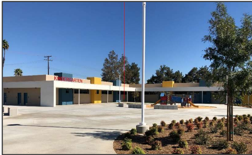
New Kindergarten Wing
