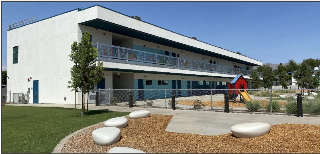
New 2-Story Classroom Building
