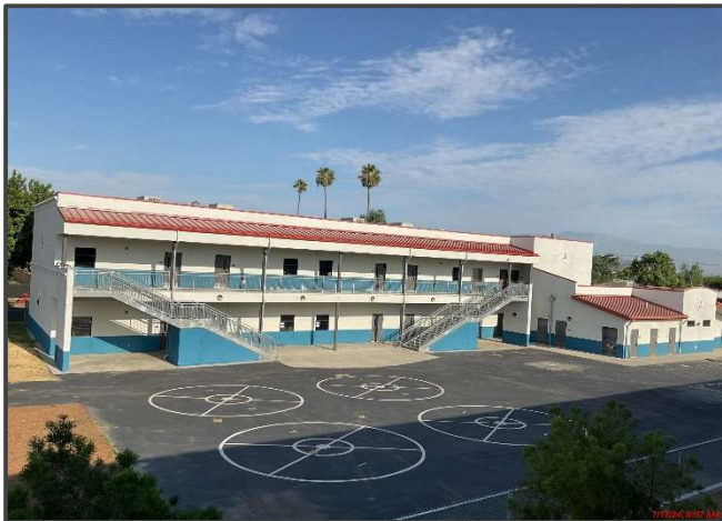
Library building repainted
