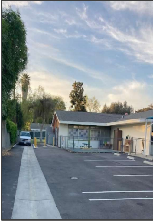
New Electrical Service
