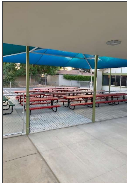
New Electrical Service
