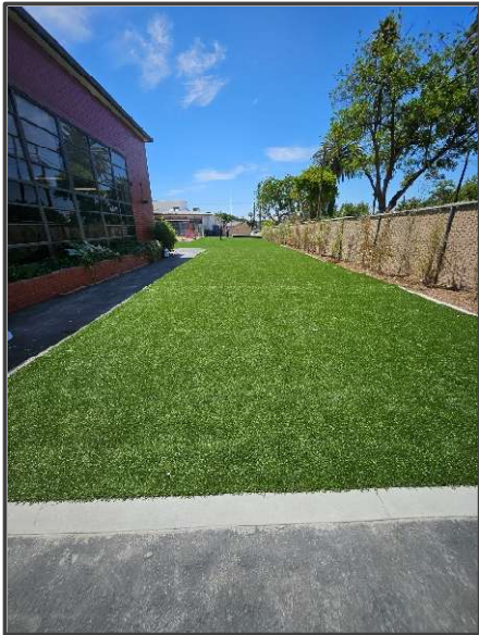
Turf Installation – Bldg. A
