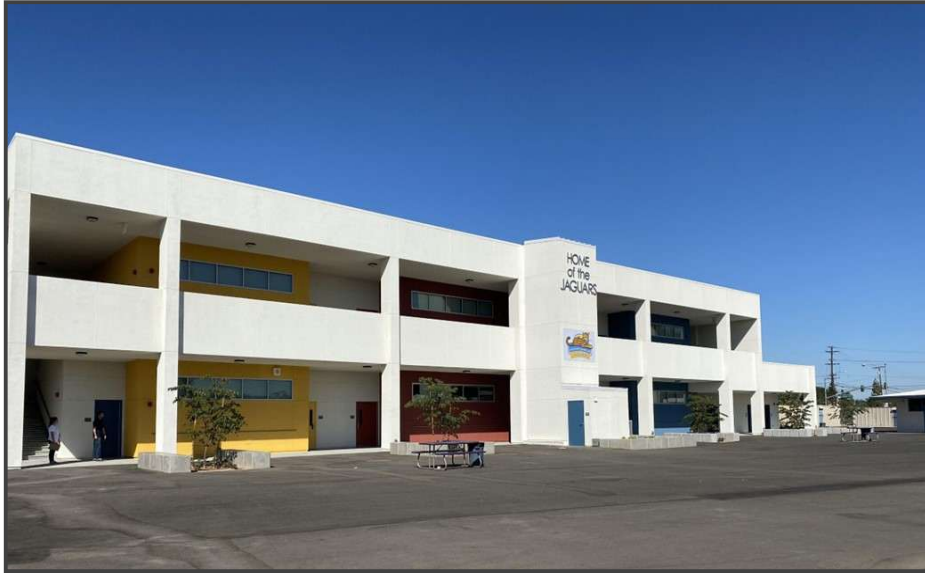
New 2-Story Building
