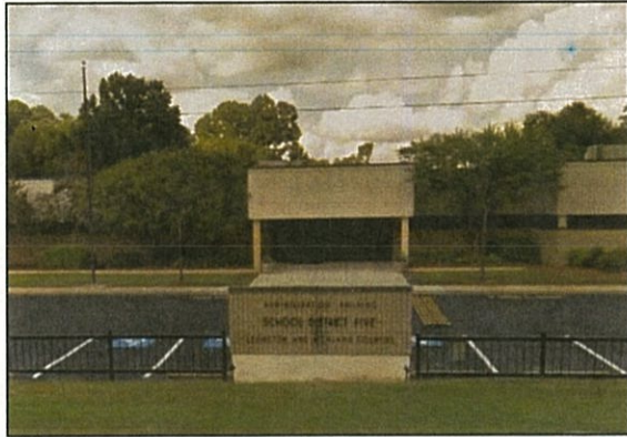
Figure 9: School District Five of Lexington and Richland Counties School District Office
