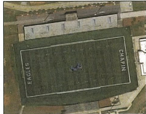
Figure 11: Chapin High School Football Stadium in need of new visitor bleachers.
