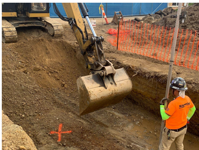
Excavation for stormwater retention system
