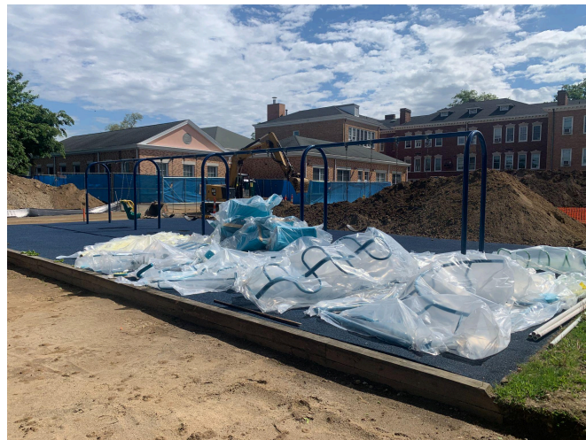
Playground equipment starting to arrive
