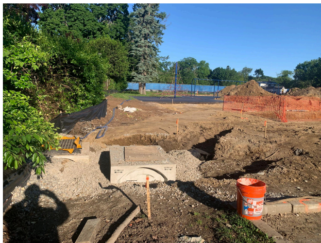
Catch basin structure installation
