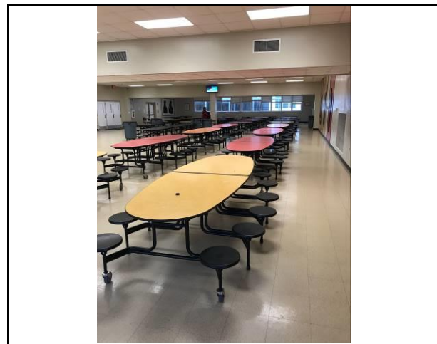
Photo #10. View of assumed vinyl floor tile ACBM in lunch room.
