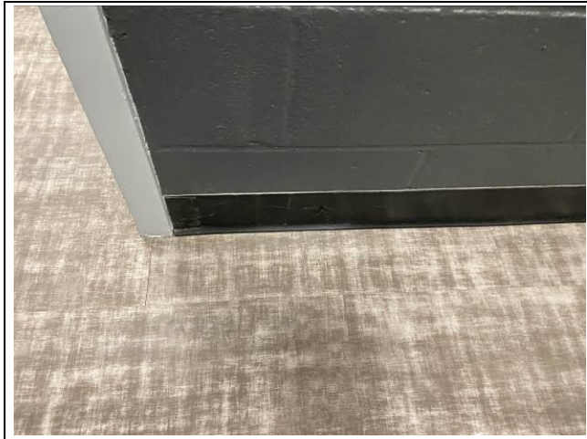
Photo #3. Typical assumed black cove base observed in the offices.
