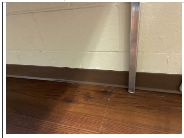
Photo #12. View of typical assumed ACBM brown cove base observed in the faculty break room.
