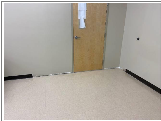
Photo #9. Another view of assumed sheetrock and joint compound form room 312.
