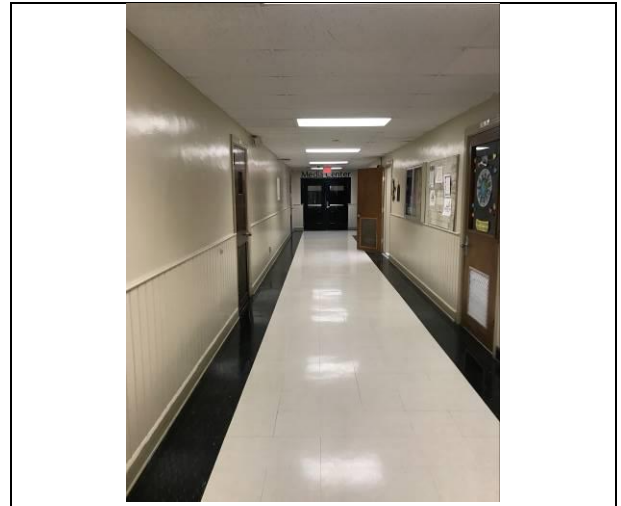
Photo #2. Typical interior finishes in History hallway.
