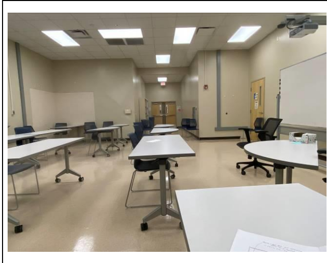
Photo #7. View of typical interior finishes observed in room 312.
