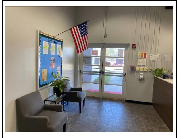
Photo #4. Typical assumed ACBM gray/white laminate flooring in the front office.
