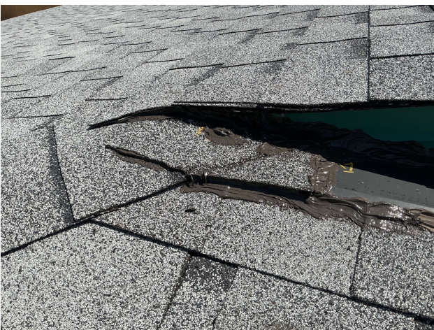
Re-installed hip cap and applied sealant for the repair
