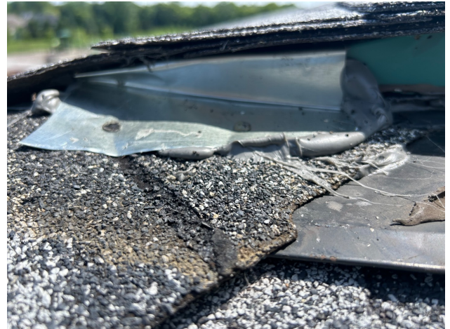
Diverter flashing installed and sealed
