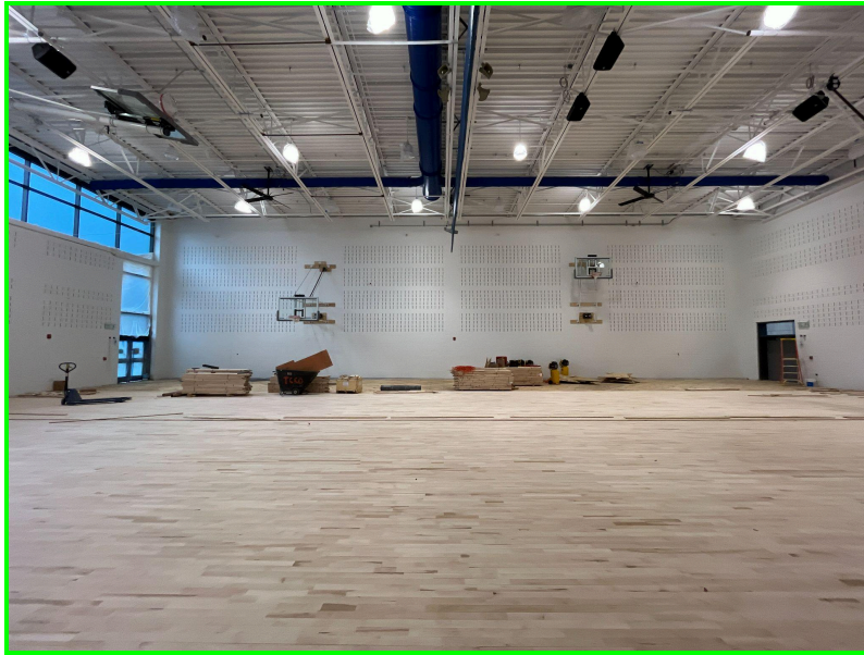
Progress photo showing installed gym equipment and ongoing installation of new athletic wood flooring
