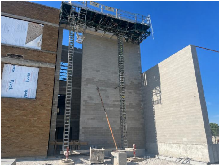
CMU Wall Stair 3 – North Side Of Area A2
