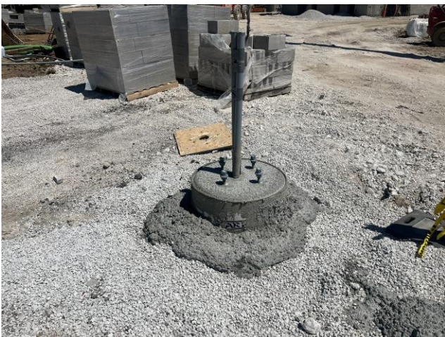
Site Light Pole Bases Installed – Playfield
