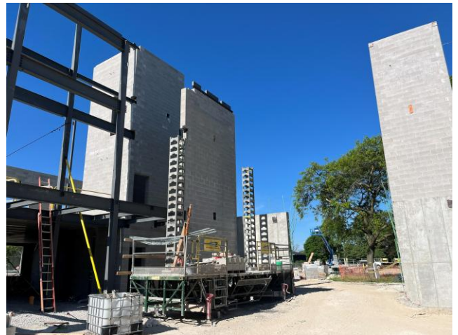
CMU Wall – Southwest Corner Of Area C1
