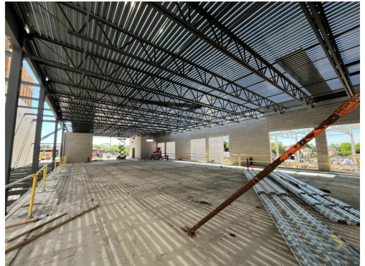
Installed Roof Decking – Area B1
