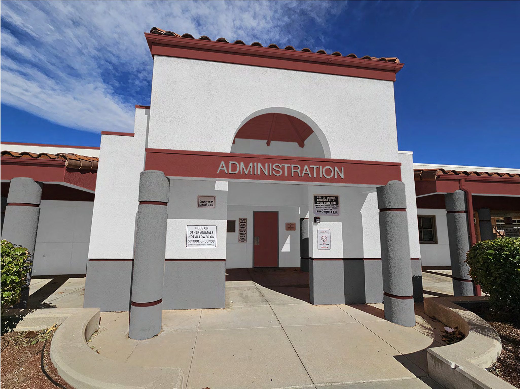
Main Entry - Administration
