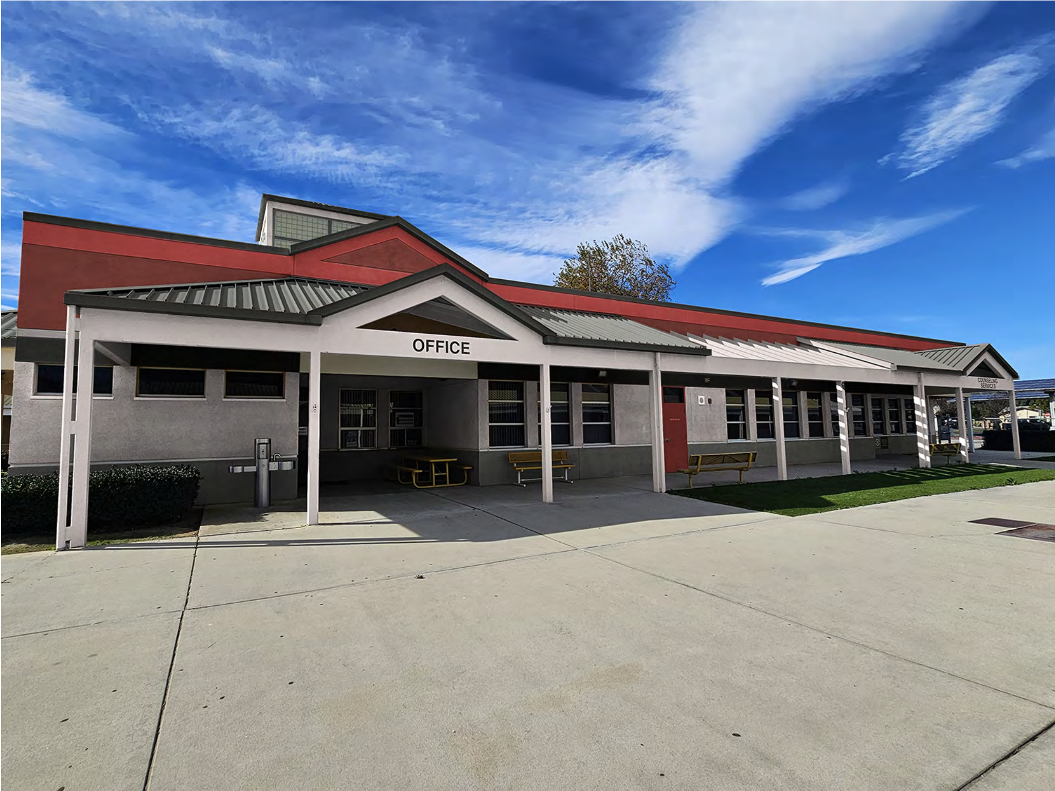
Administration (East Face)
