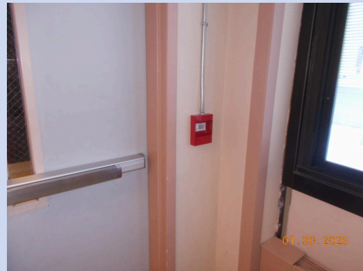
New fire alarm pull station at School One.
