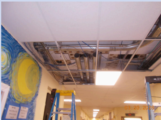
New electrical service piping being added at
