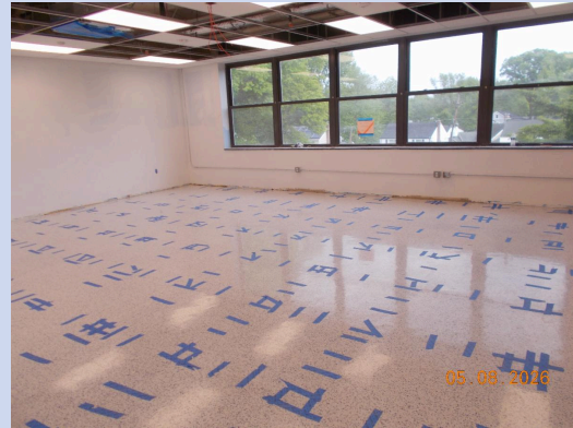
La Grande second floor classroom flooring installation.
