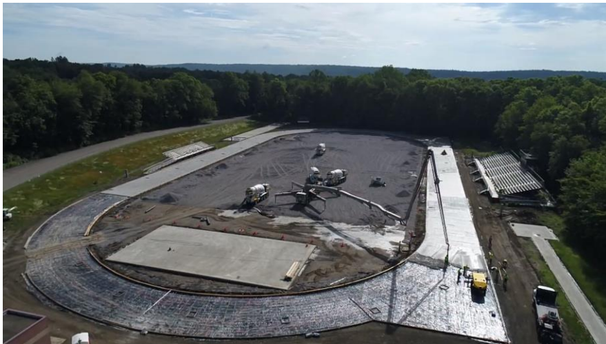
TRACK AND FIELD CONSTRUCTION 2021
