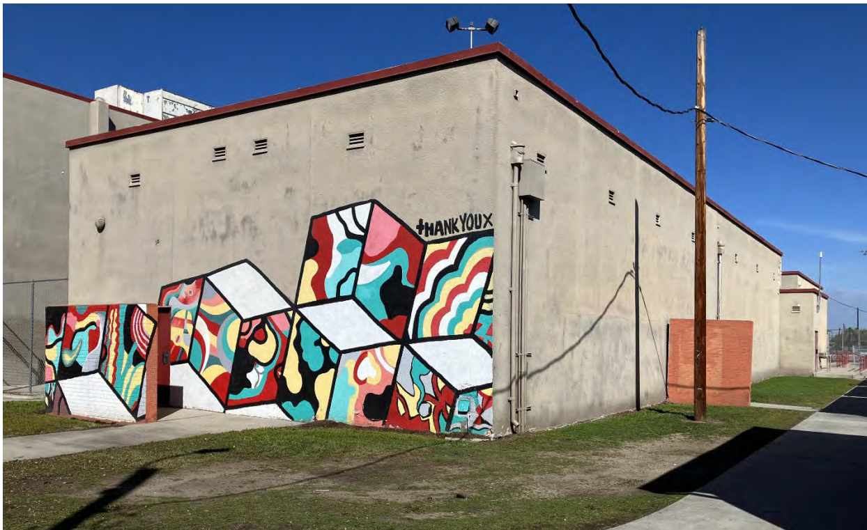
Photo 6. Unit R – Girls' locker room, west and south facades, looking northeast. Ascent 2025.
