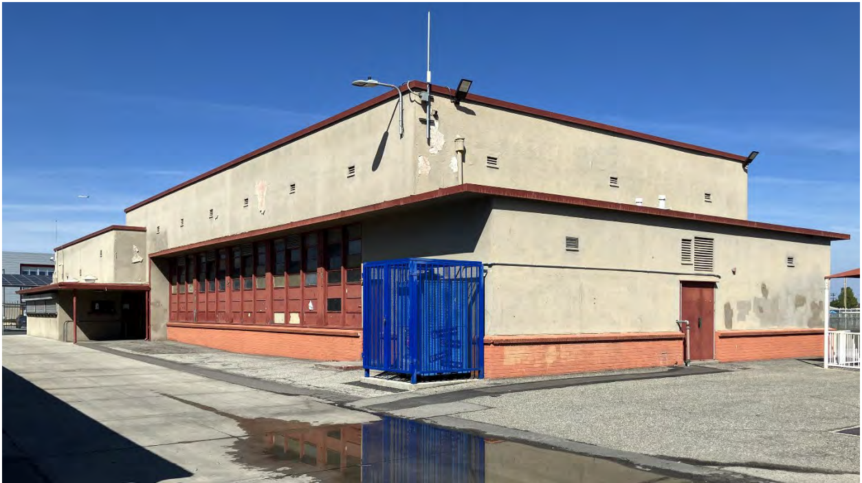
Photo 10. Cafeteria, west and south façades, looking northeast. Ascent 2025.
