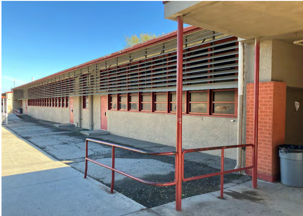
Photo 14. Unit BB, north façade, looking northwest, representative of 1960s classroom. Ascent 2025.
