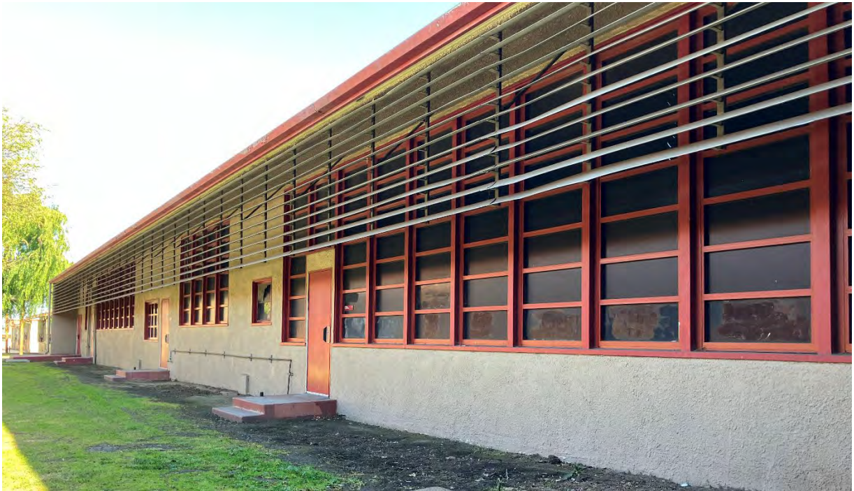
Photo 12. Unit K, north façade, looking southeast, representative of original classroom buildings. Ascent 2025.
