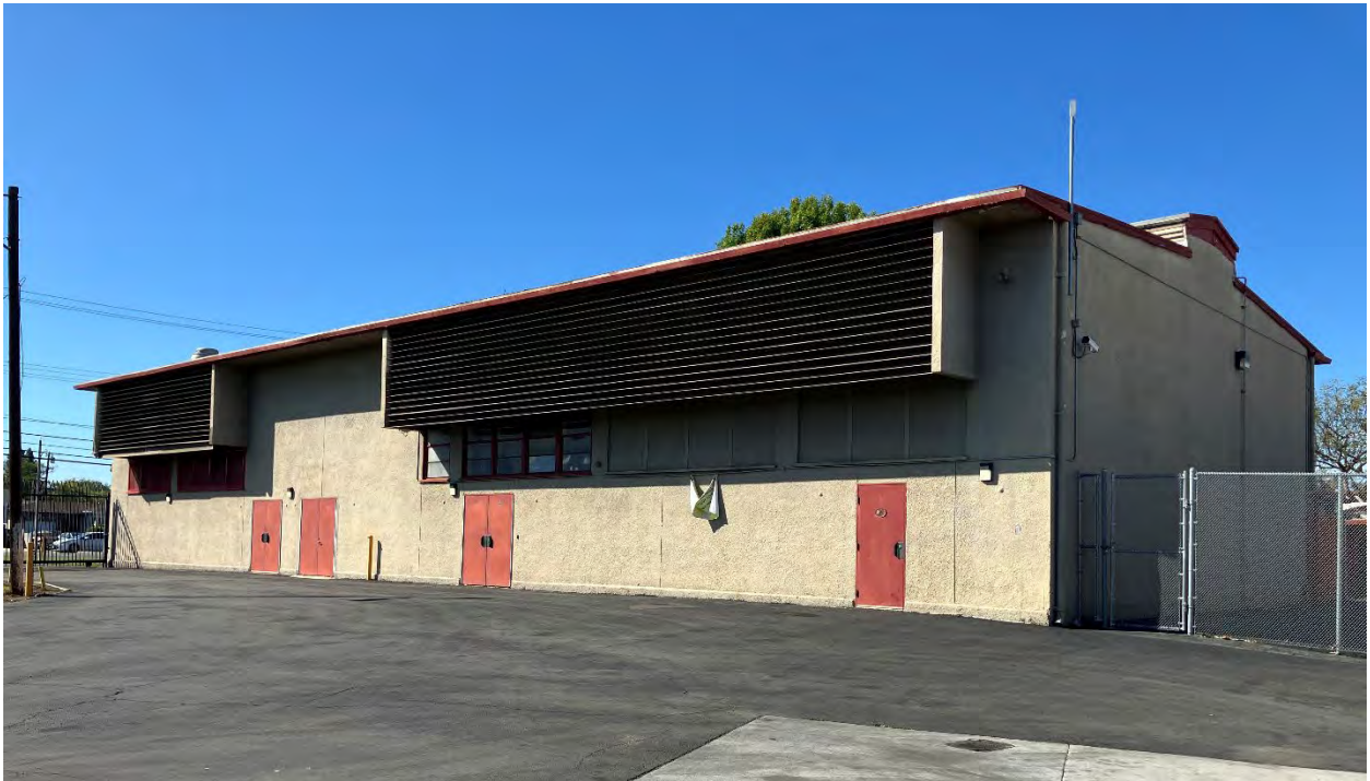
Photo 16. Unit M, south and east façades, looking northwest, former woodshop. Ascent 2025.
