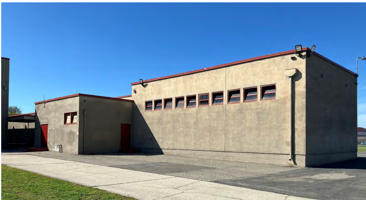
Photo 7. Unit Q – Boys' locker room, east and north facades, looking northwest. Ascent 2025.
