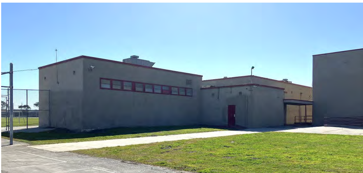
Photo 5. Unit R – Girls' locker room, east and north facades, looking southwest. Ascent 2025.
