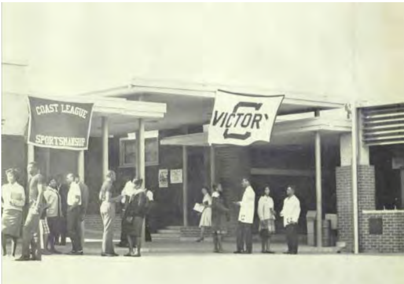
Figure 16. 1962 yearbook. Administration Building/Library east facade, looking northwest.
