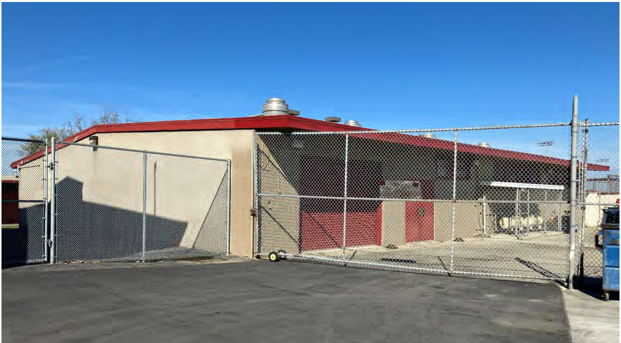
Photo 17. Unit N, west and south façades, looking northeast, auto shop. Ascent 2025.
