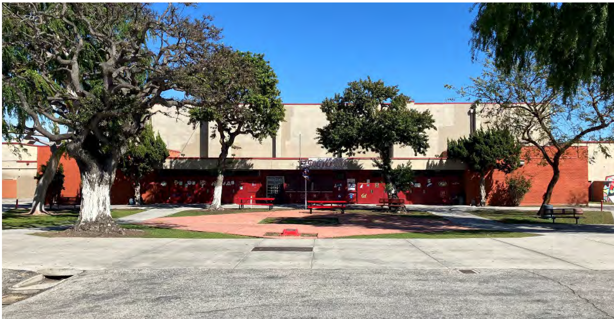
Photo 4. Gymnasium with Senior Square in the foreground, west façade. Ascent 2025.
