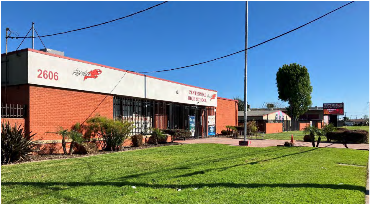
Photo 2. Left to right - Administrative Building/Library, Unit DD, Unit L, and Unit M. West facades fronting N. Central Avenue. Ascent 2025.
