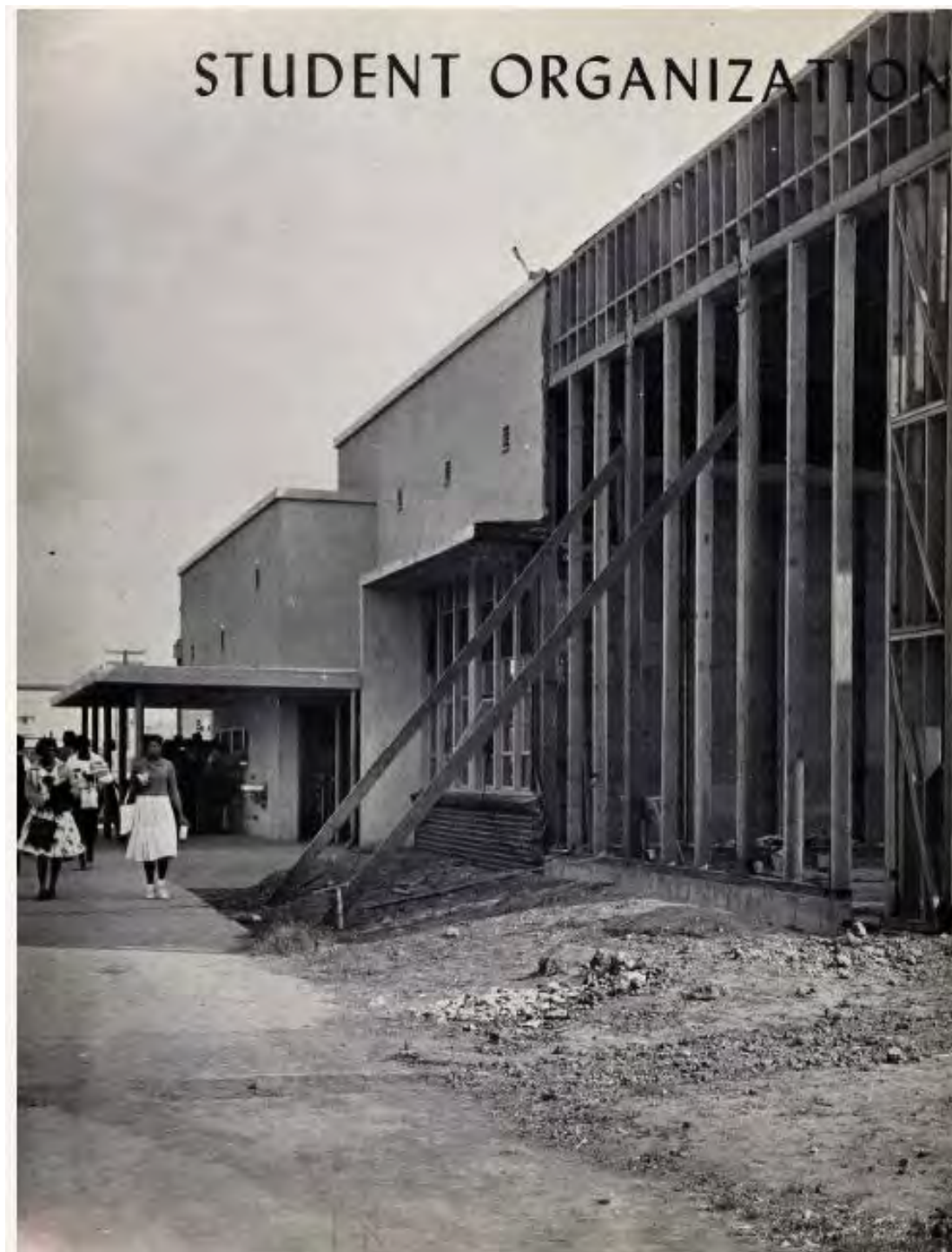
Figure 14. 1961 yearbook. Cafeteria expansion, looking north.
