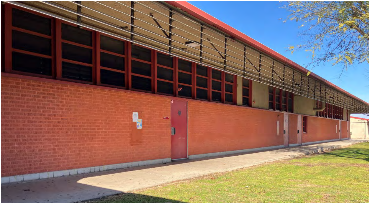
Photo 11. Unit K, south façade, looking northeast, representative of original classroom buildings. Ascent 2025.
