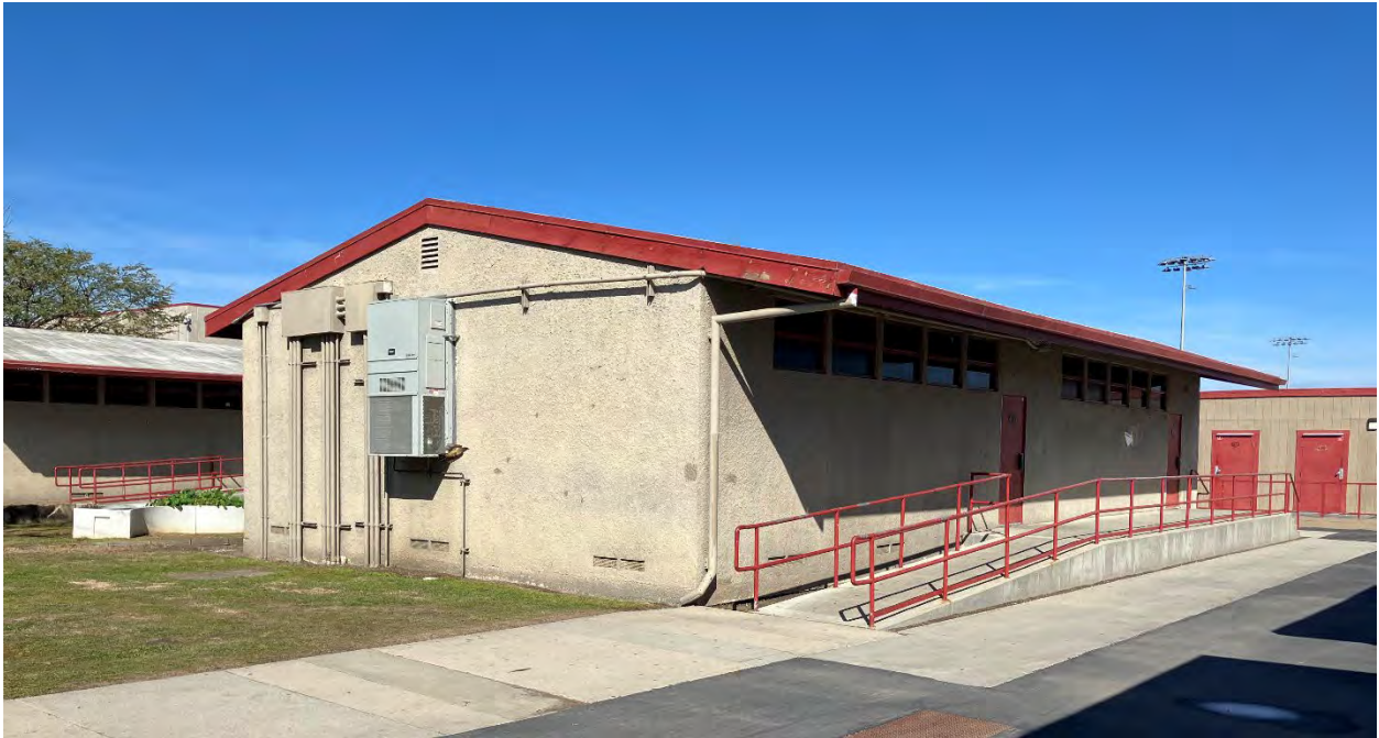
Photo 15. Unit Y, west and south façades, looking northeast, representative of a small classroom building. Ascent 2025.
