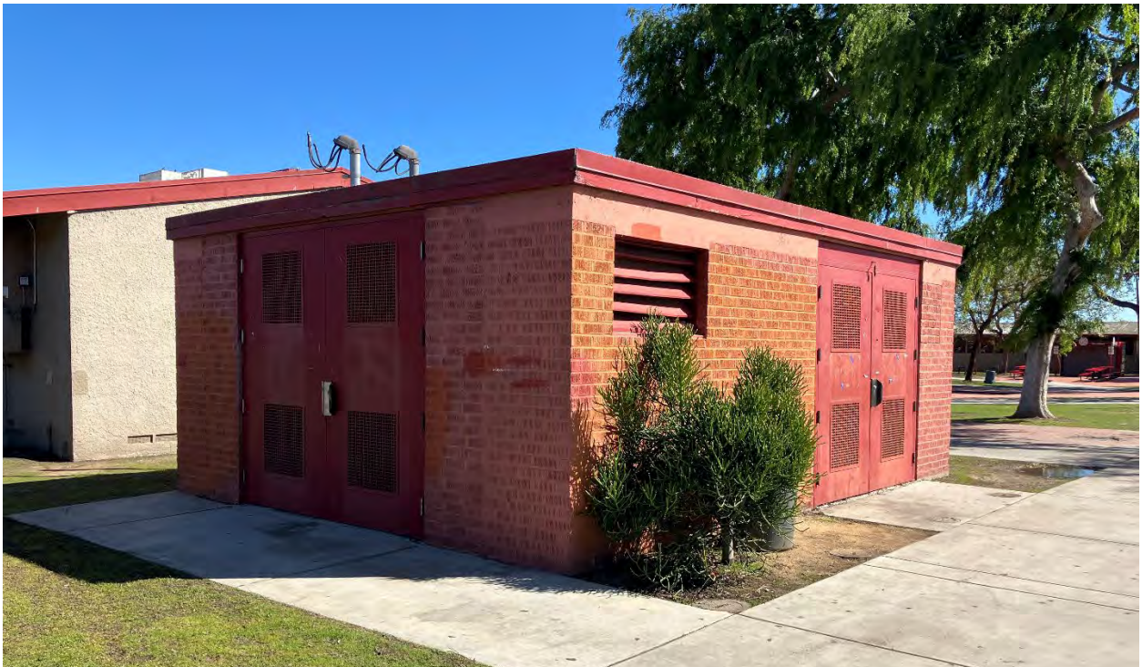
Photo 9. Unit P – utility building, north and west façades, looking southeast. Ascent 2025.
