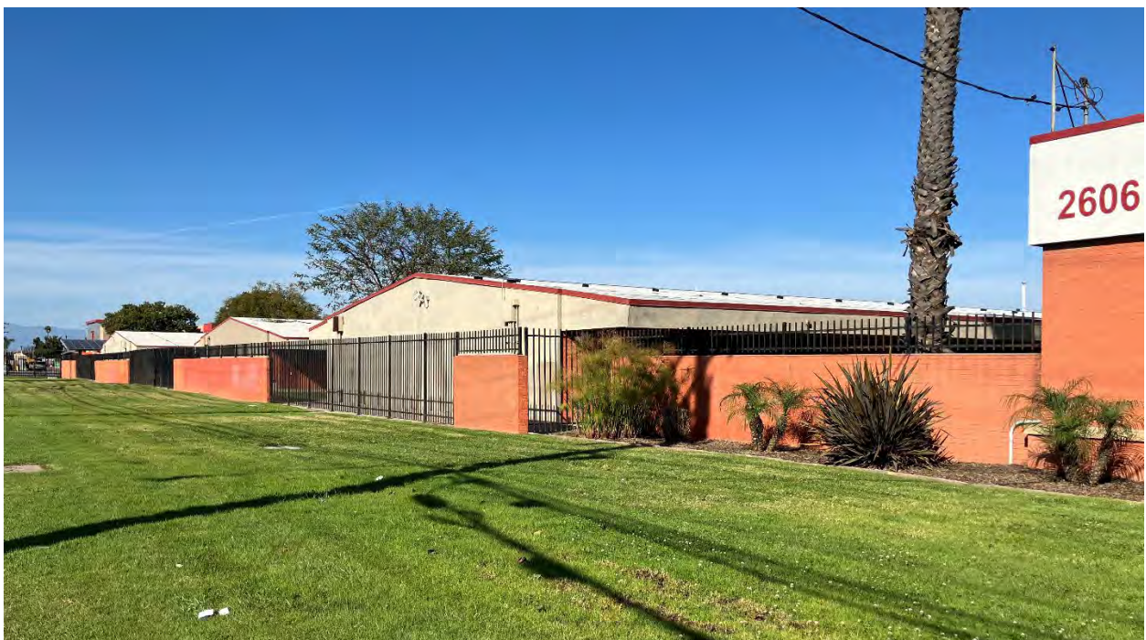
Photo 3. Left to right – Unit AA, Unit BB, and Unit CC. West facades fronting N. Central Avenue. Ascent 2025.
