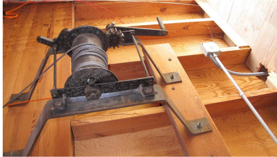
Reference Photo 2 - Two Rivers-Dos Rios Elementary: Basketball hoop cable hoist can be removed and reinstalled as required to allow for end anchorage installation.
