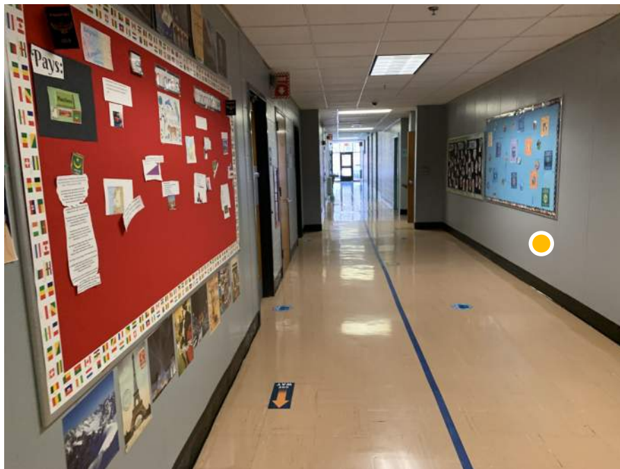
● D1. 66: View of typical corridor in 1972 addition, note the modular wall construction.
