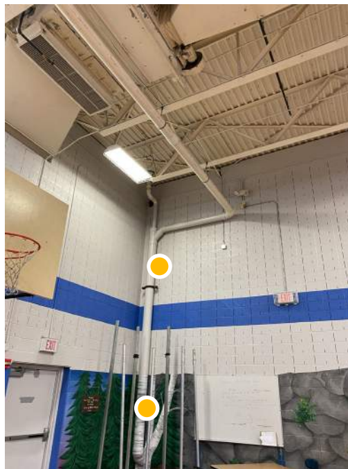
● D2. 52: detail view of exposed piping in auxiliary gymnasium.
