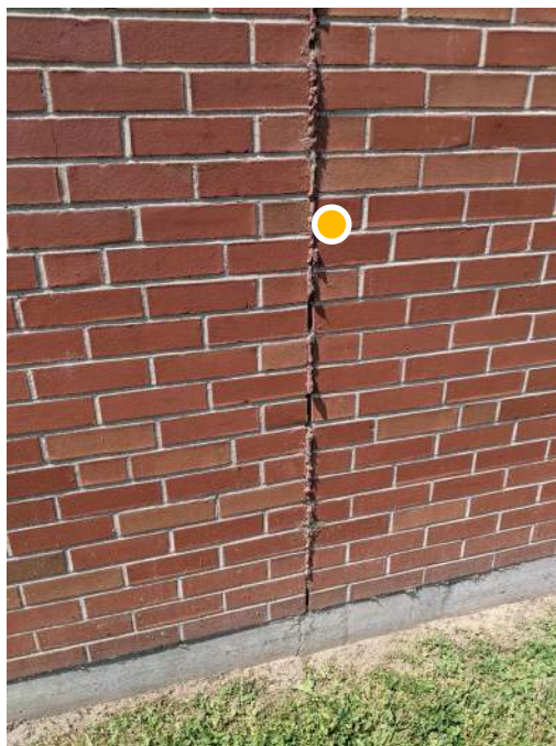
● D1. 17: Detail view of typical expansion joint in poor condition overall.
