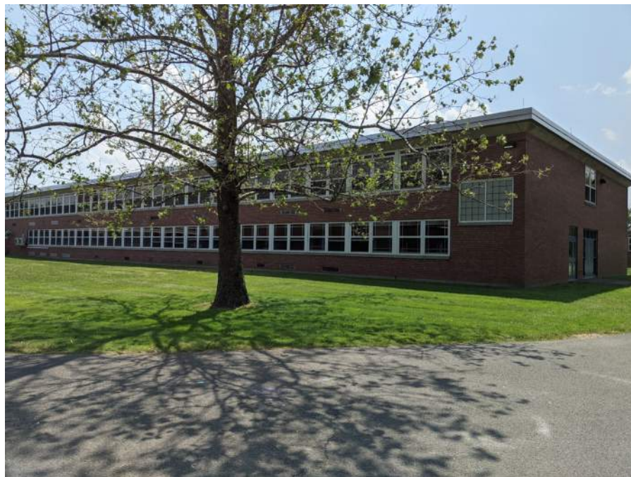
● D1. 24: Overall view of the two story classroom portion of the middle school, original construction 1964.
