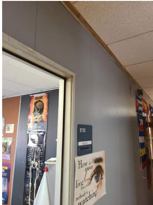
● D1. 43: Detail view of modular wall construction in the 1972 addition
