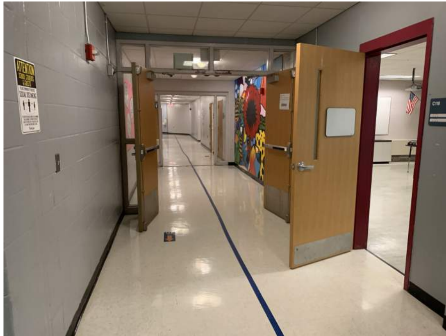
● D1. 71: View of typical corridor in original 1964 building.
