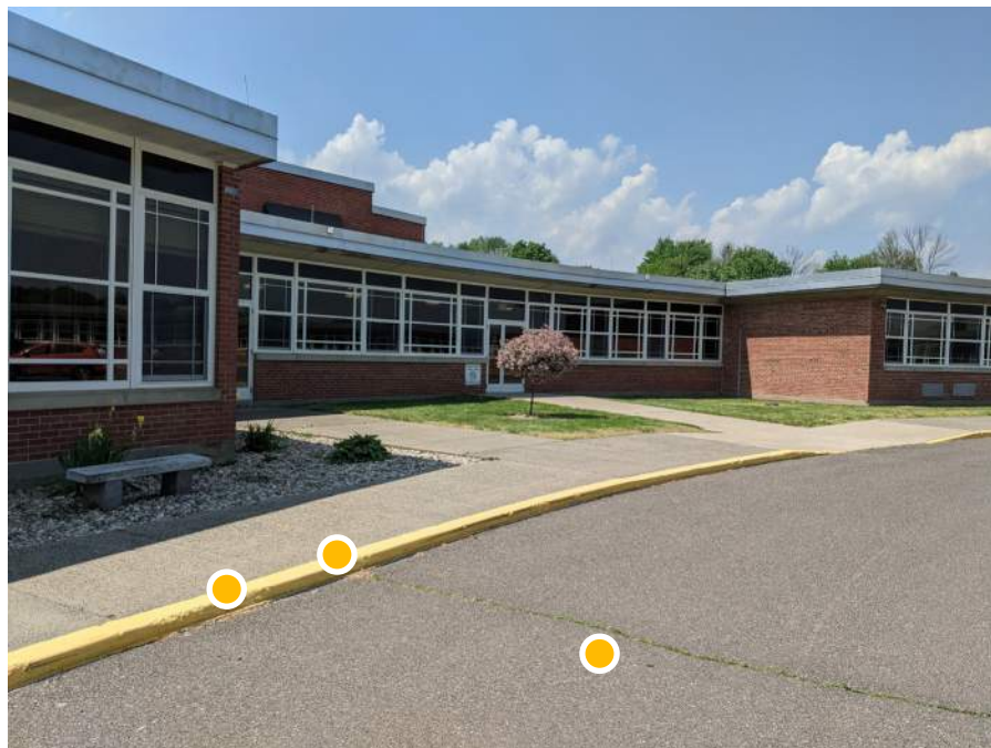
● D3. 4: View of courtyard between existing auditorium and classroom wing.
