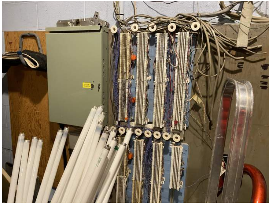
● D2. 59: Telephone Service Distribution.
