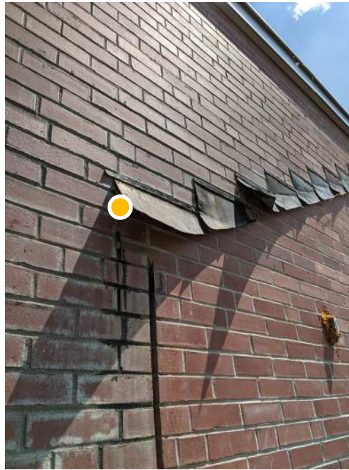
● D1. 23: Detail view of the step flashing that remains from the former greenhouse, part of the 1965 Vo-ag addition.
