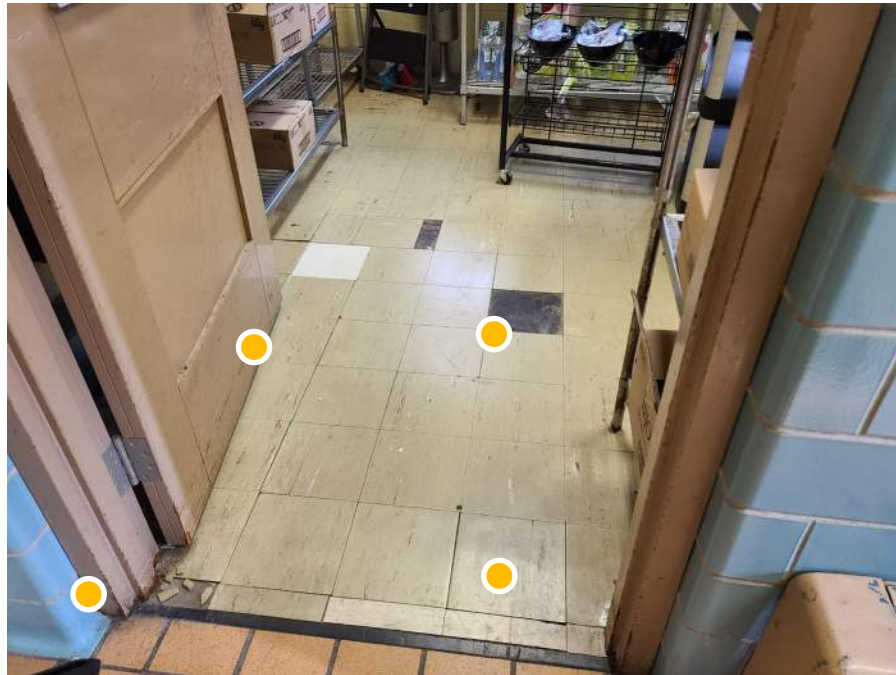
● D1. 51: Detail view of dry storage support space for the cafeteria, note the poor condition of the door, door frame and flooring.
