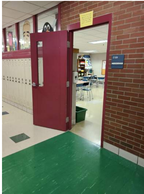
● D1. 55: Typical entry door into classrooms
