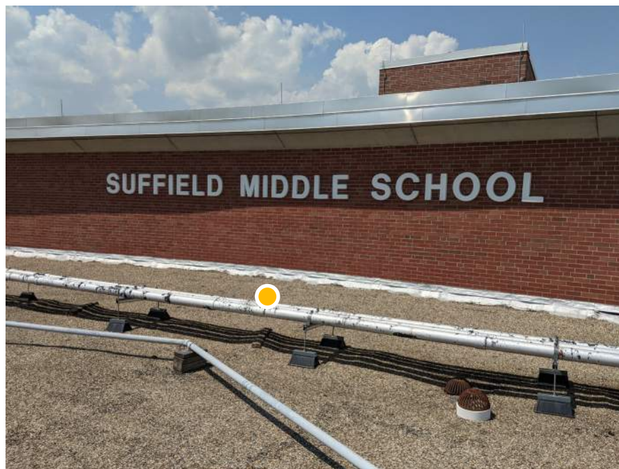
● D1. 12: Detail view of original 1964 construction, two story portion, with surface mounted electrical conduits, roof mounted, into original electrical room.
