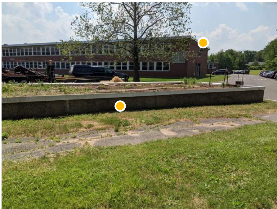
D3. 2: View of former greenhouse foundation wall in foreground, two story classroom wing shown beyond.
