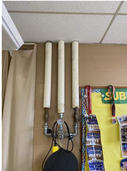
● D2. 11: Domestic Water Thermostatic Mixing Valve.
