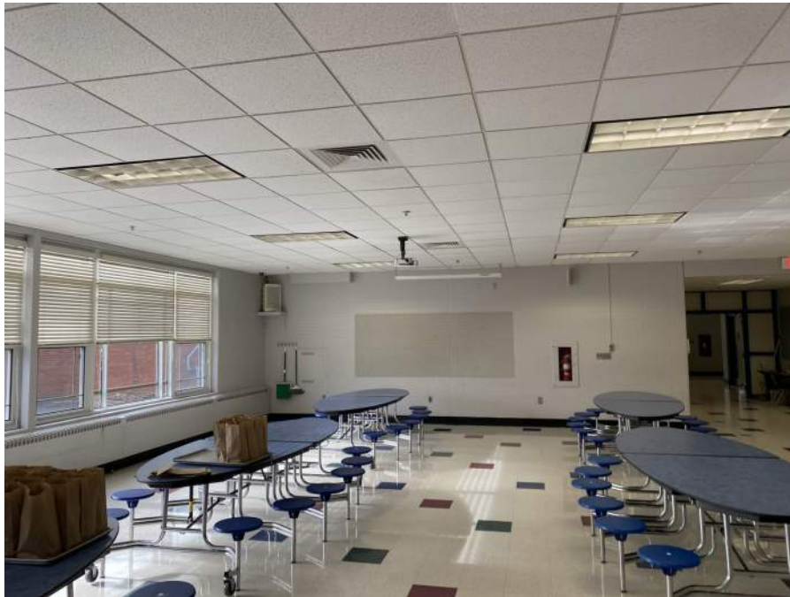
● D2. 41: View of existing cafeteria, original construction 1964.
