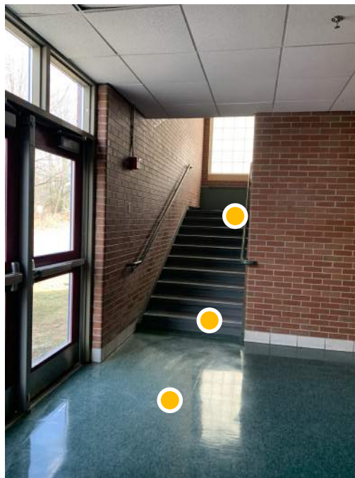
● D1. 72: View of retrofit and upgrades to the north egress stair in original building
