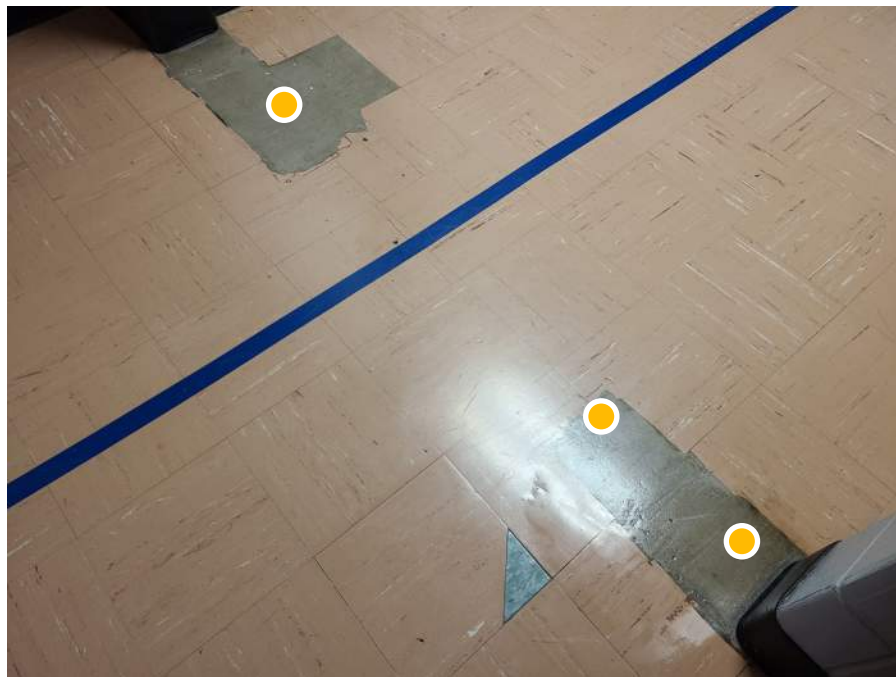
● D1. 48: Detail view of flooring patch/retrofit, possible vinyl asbestos tile original to building.
