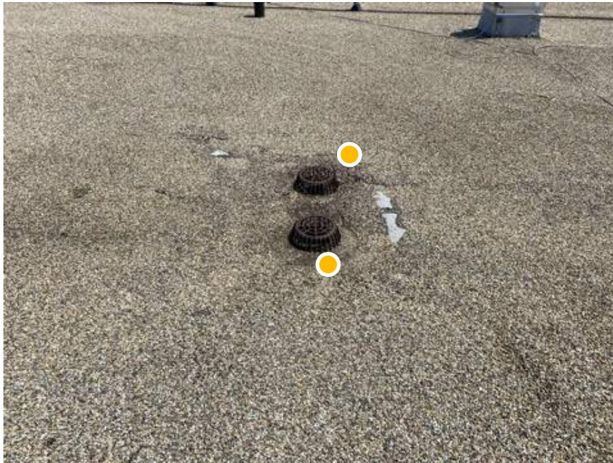
● D2. 53: View of typical roof drain.
