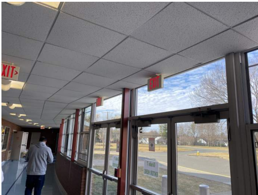
● D2. 42: View of entry vestibule area adjacent to the gymnasium, original construction 1964.
