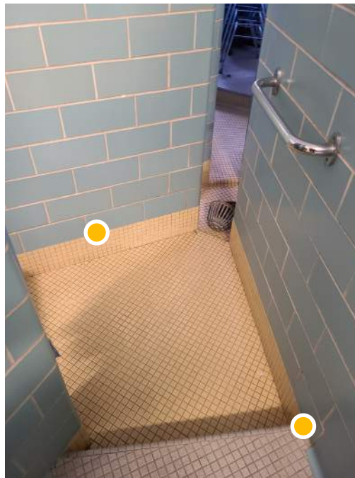
D1. 34: View of girls shower stall in original building, no longer utilized and does not meet current accessibility codes.
