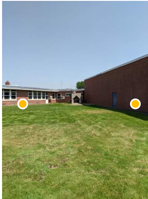
● D3. 3: View of courtyard between existing auditorium and classroom wing.
