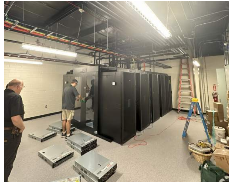
Data Pod Install
