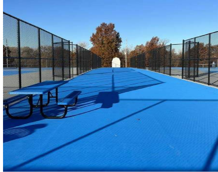
Center Spectator Concourse Looking West
