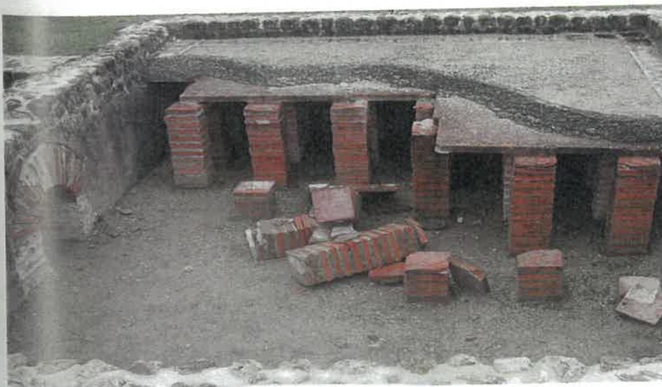
A Roman hypocaust (underfloor heating system). On the left you can see where the hot air would have flowed through from the furnace.
