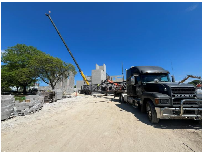
Long Span Joist Delivery – Area C2
