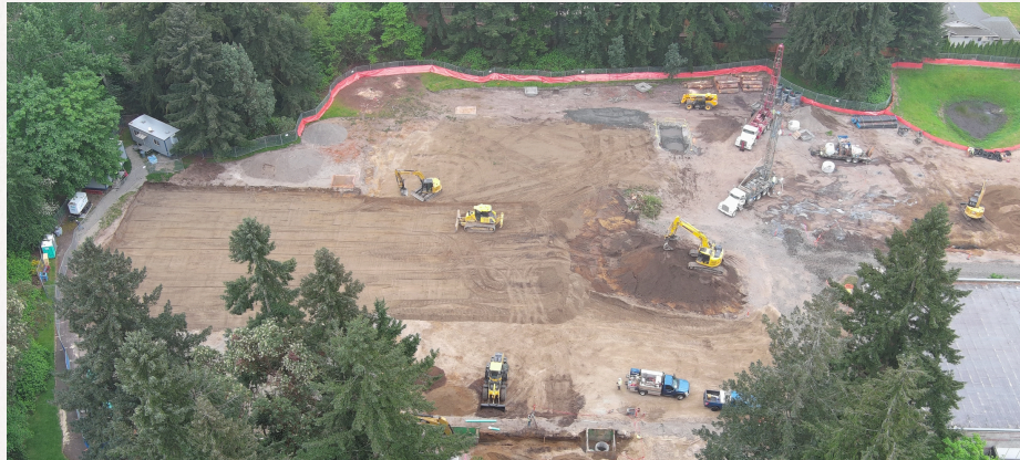
Photo looking South from above existing building
