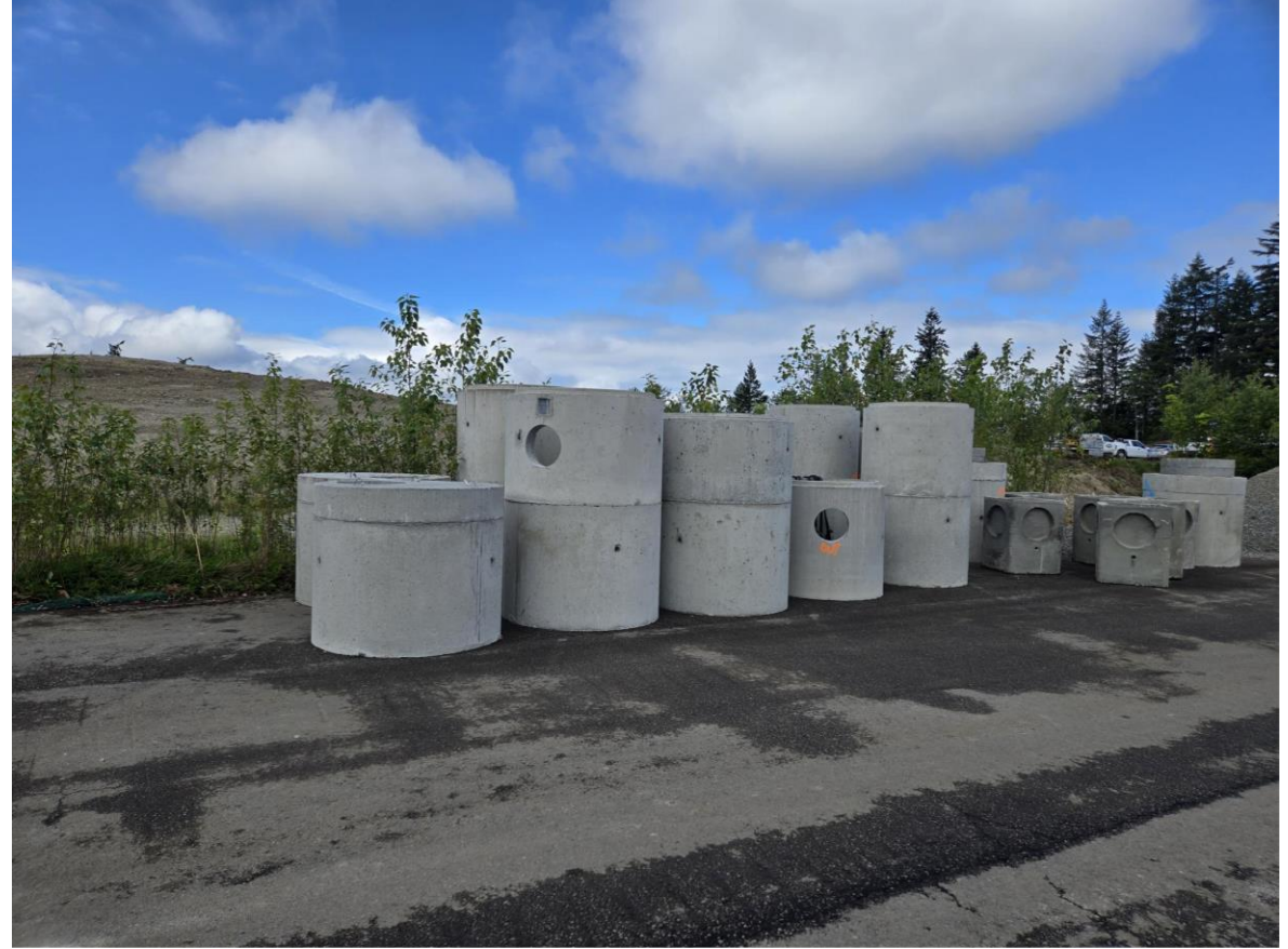
Storm water structures be stockpiled on the site
