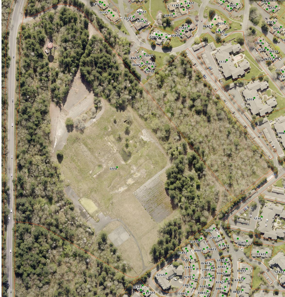
Site before construction started
