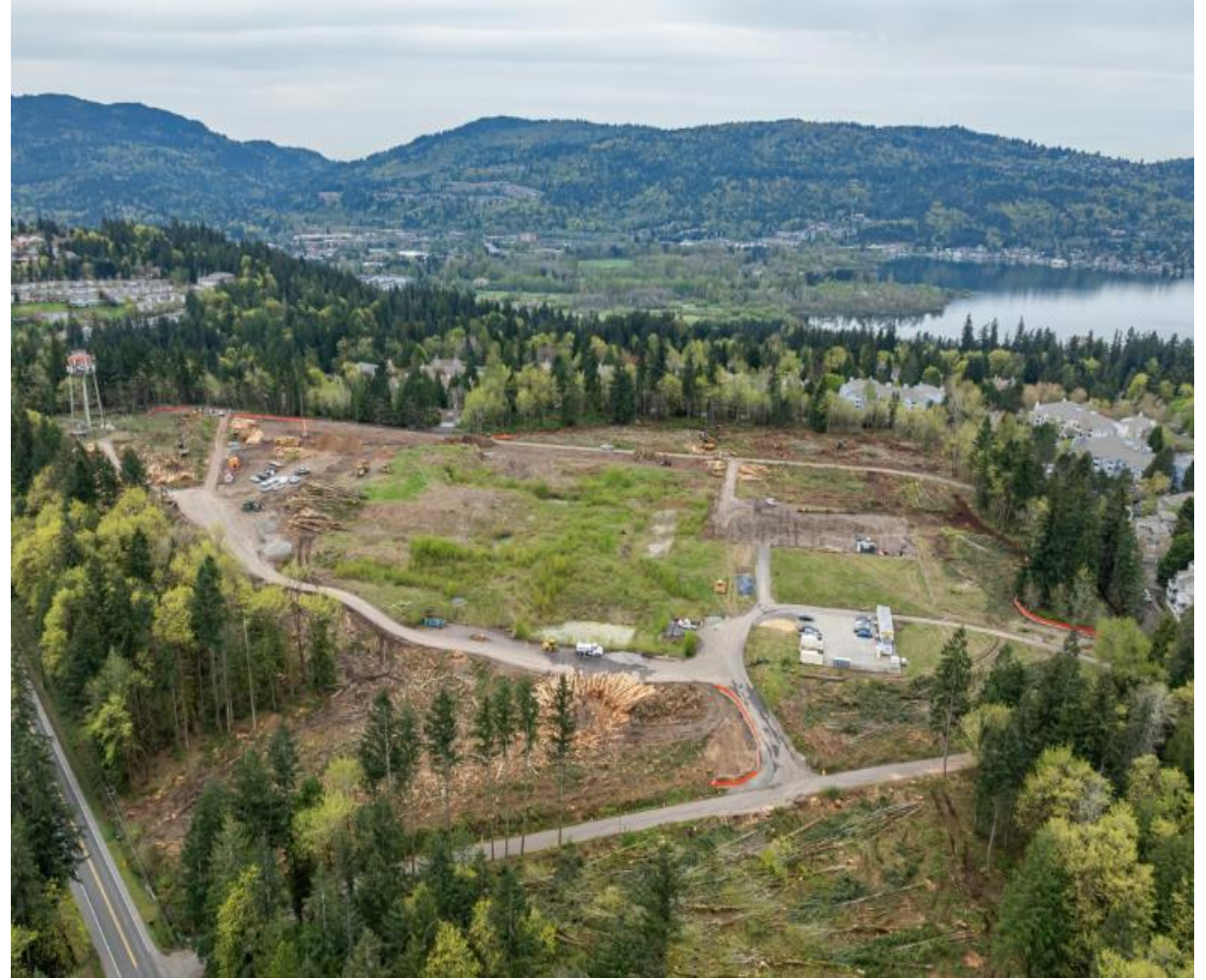
Site cleared and ready for grading
