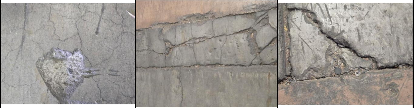
Building W - Stair Carpet & Mastic
