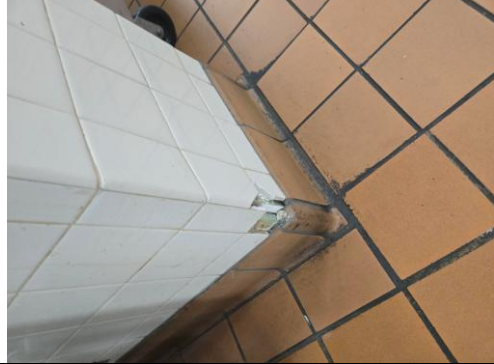
2" x 2" Ceramic Floor Tile, Grout, & Mastic
