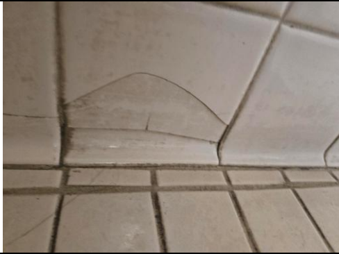
Marble Threshold & Mastic
