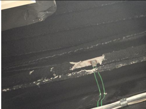
Black Foam Pipe Insulation
