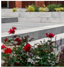
CONCRETE STEPS AND RAMPS
