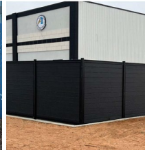
BOARD FENCE (LIBRARY/LOADING)
