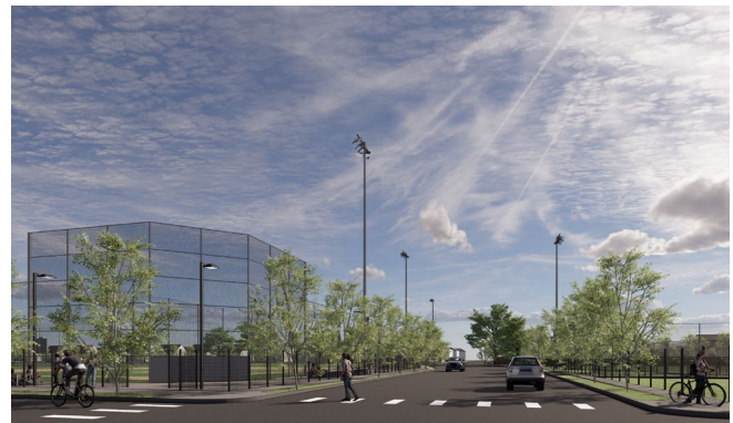
Intersection of Alberta and Kerby
