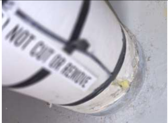
White Pipe Wrap, Yellow Insulation, & Mastic
