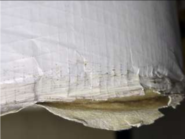
White Pipe Wrap, Yellow Insulation, & Mastic
