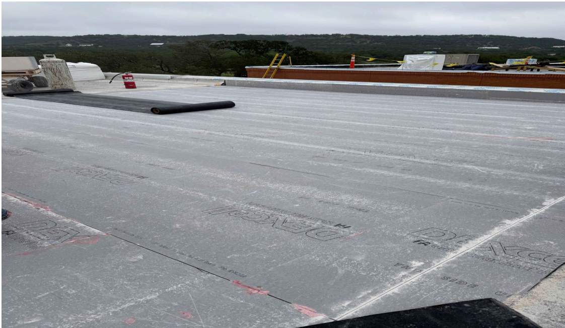
Photo: Roof Replacement at Blue Hole
