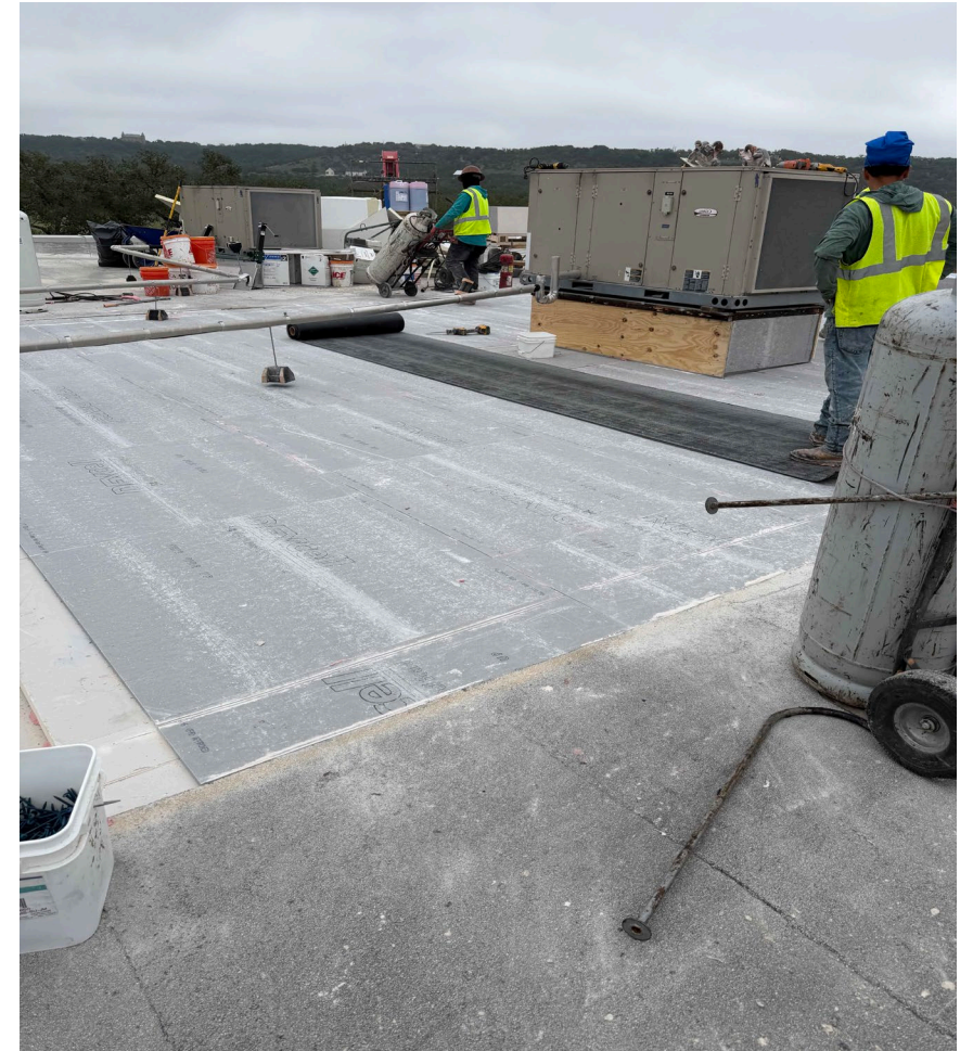
Photo: Roof replacement at Blue Hole
