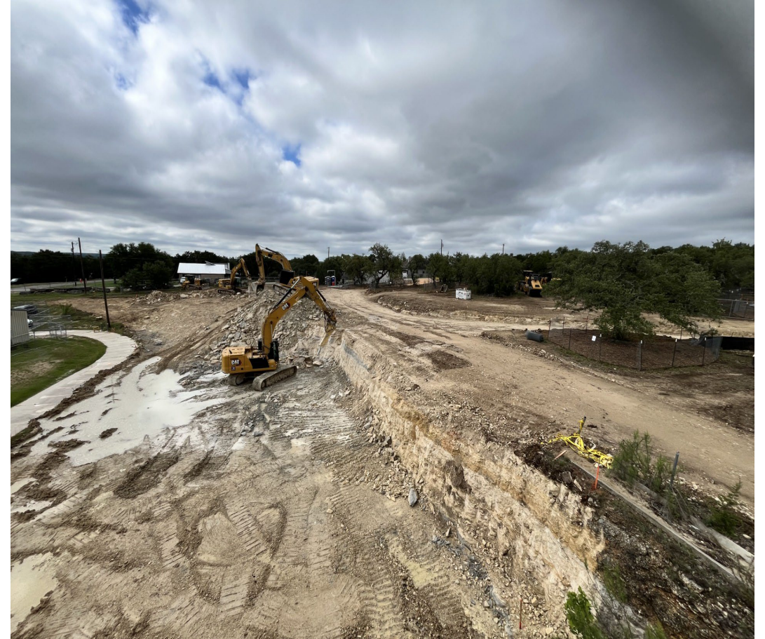
Photo: Band Marching Pad Retaining Wall
