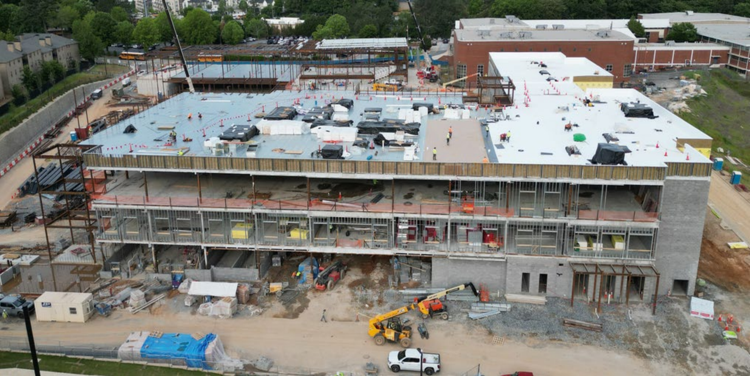
Area '4' External Metal Framing
