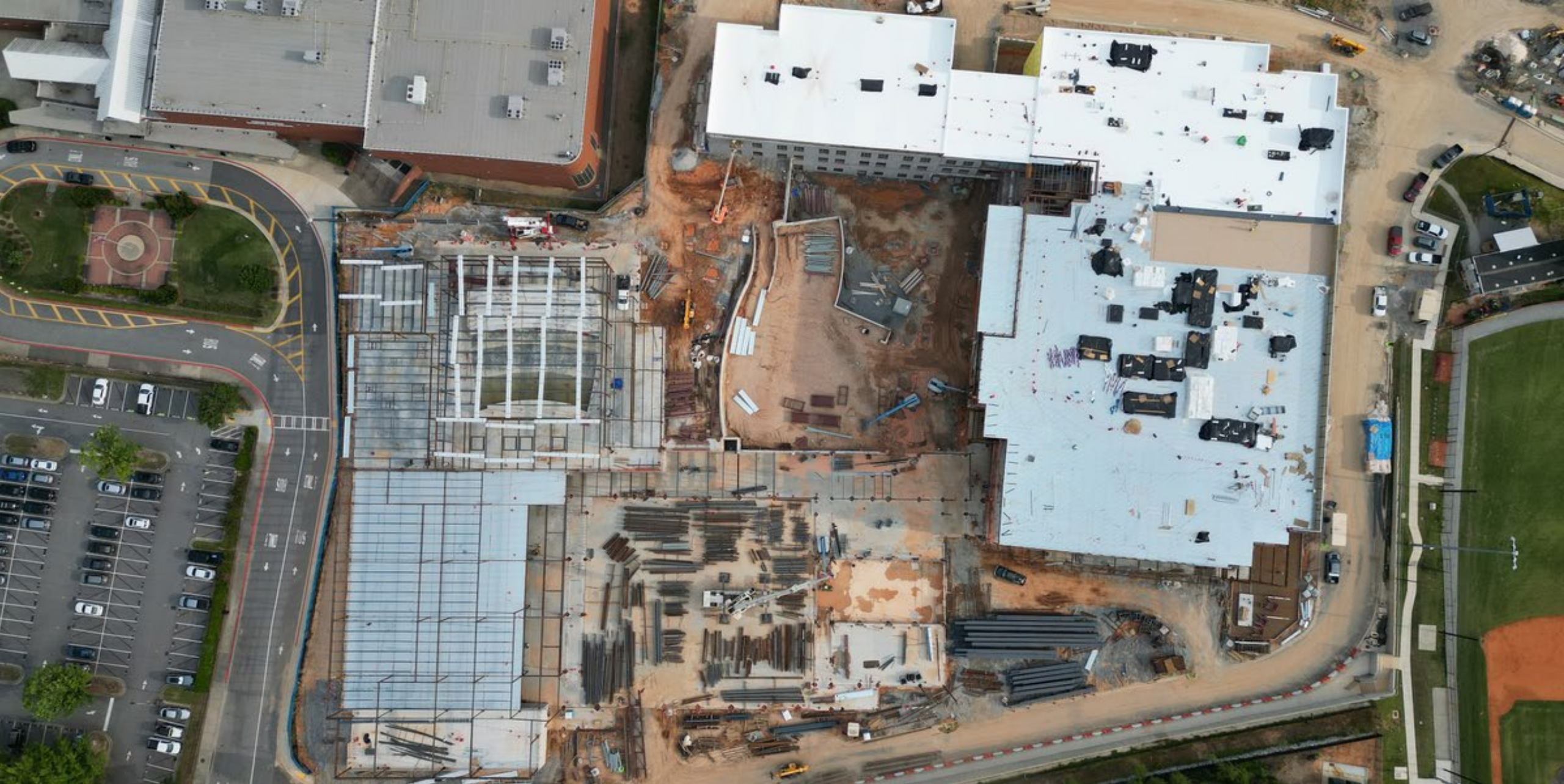
Overall Site Progress
