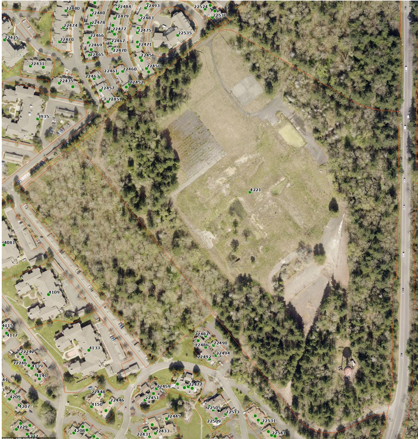
Site before construction started
