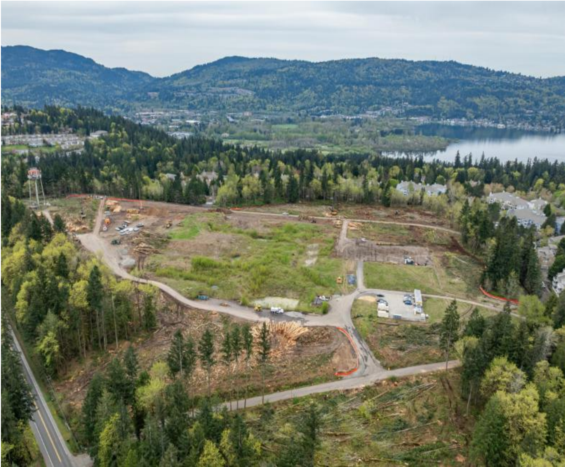
Site cleared for grading
