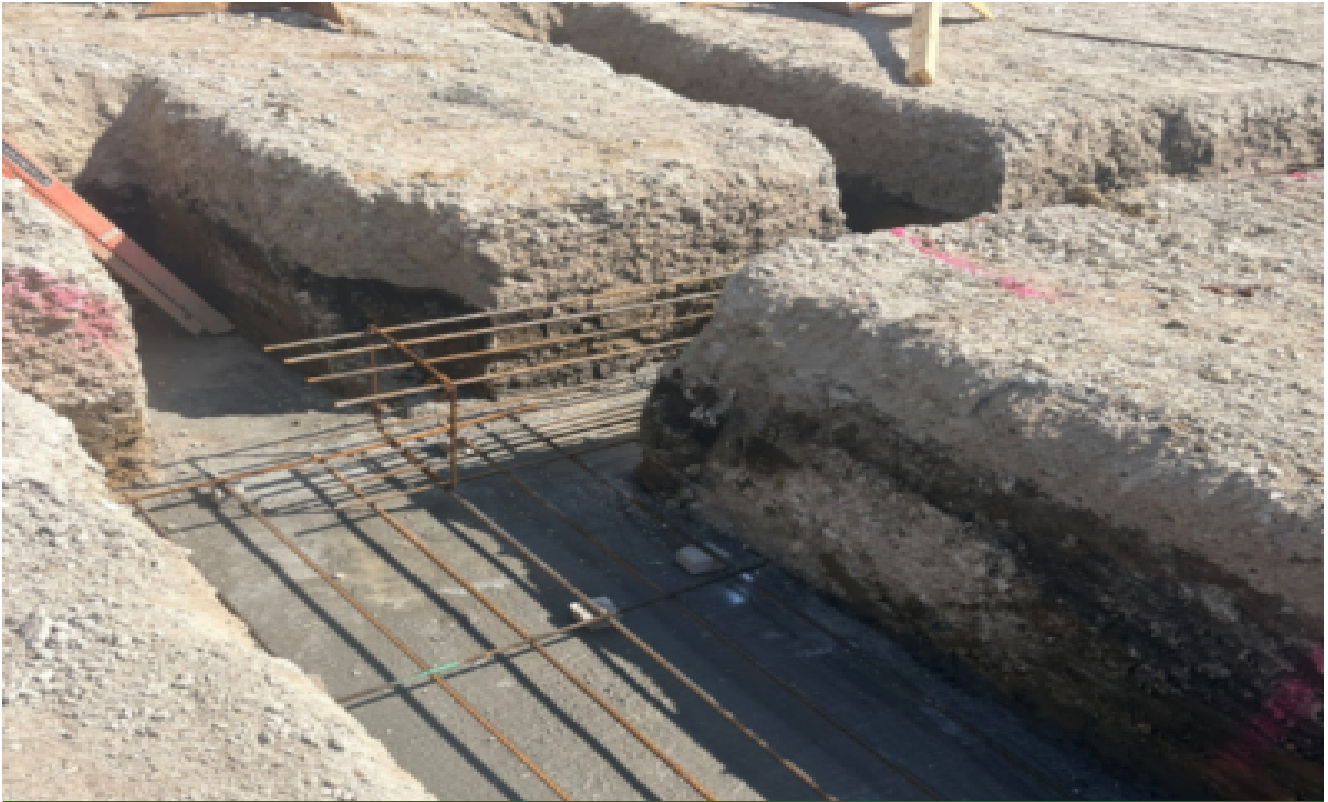
Preparation of Area B Foundations
