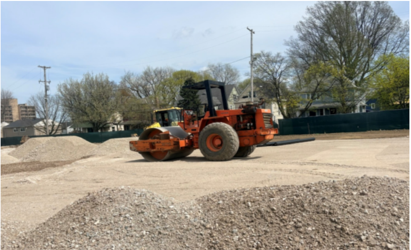
Building Pad, Remediation
