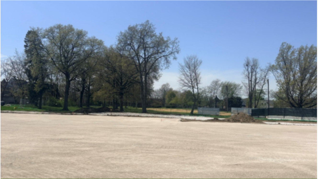
Building Pad, Completion of the Remediation
