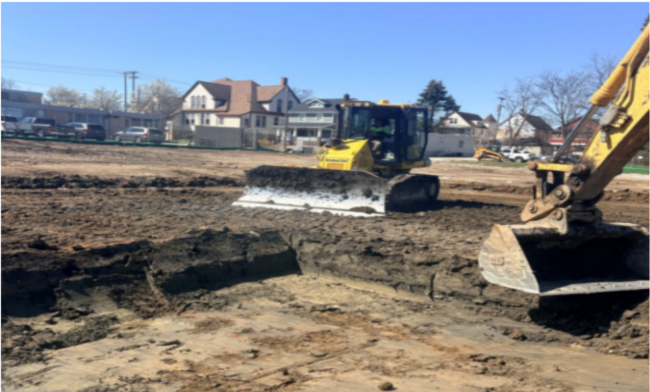
Building Pad, Undercut
