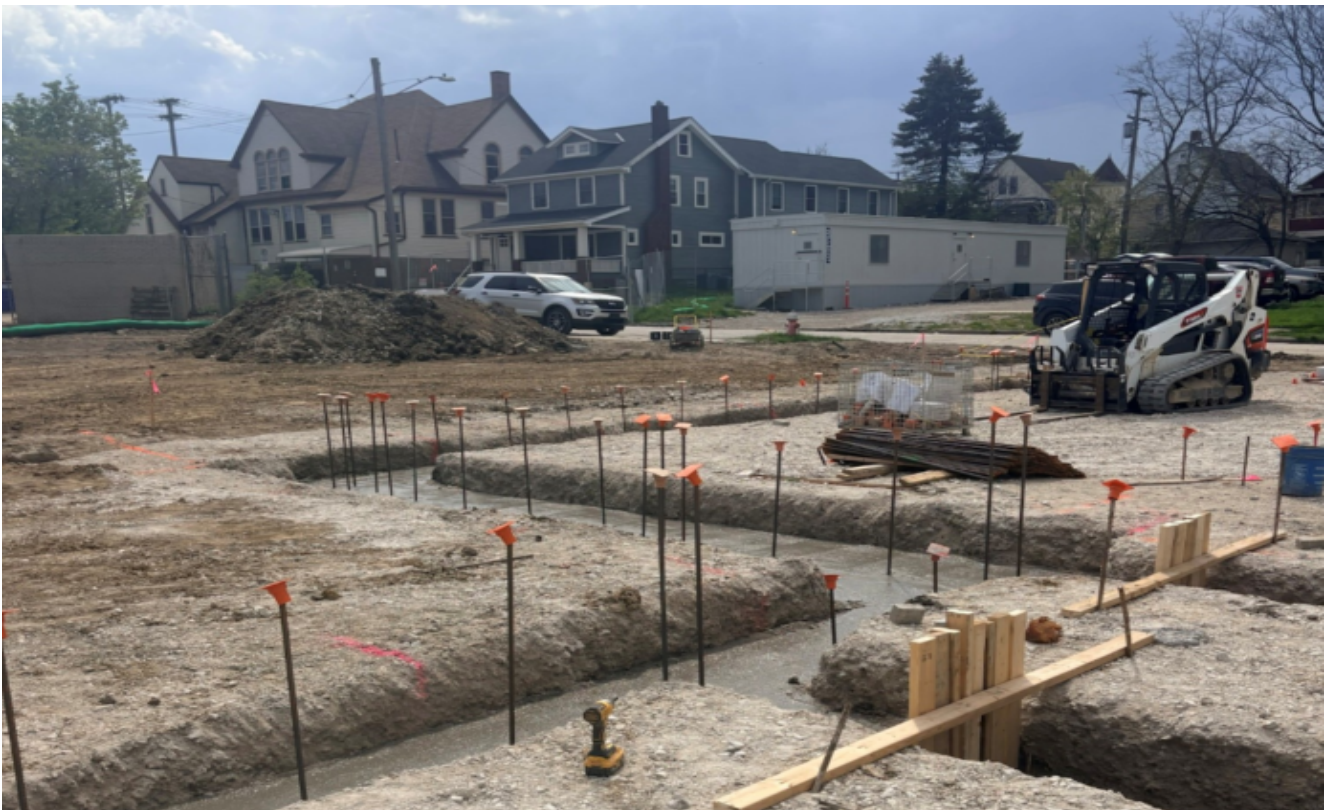
Area B Concrete Foundations
