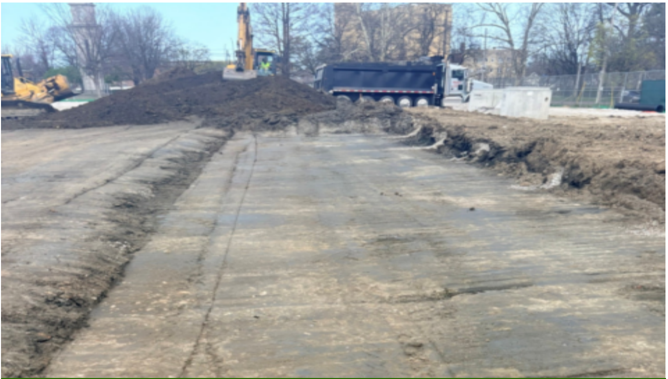
Building Pad, Undercut
