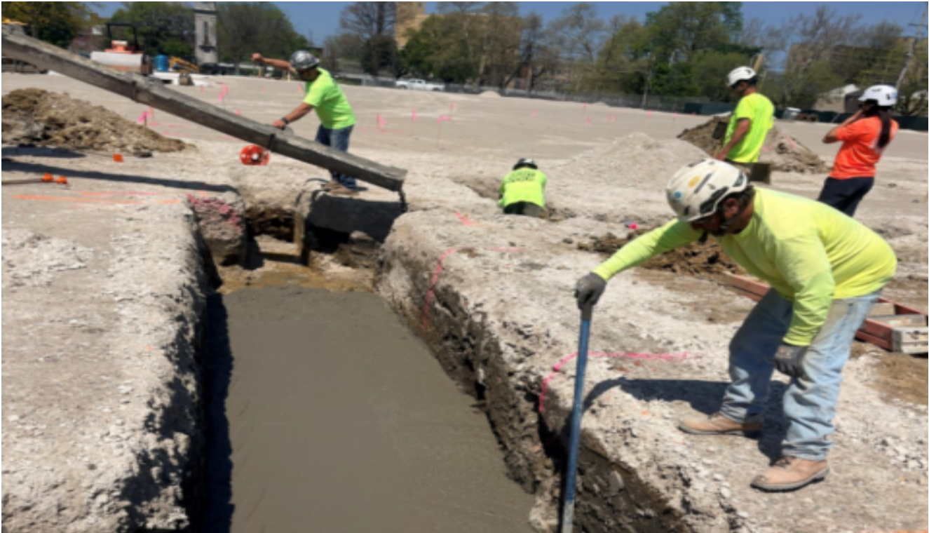
Placement of Concrete for Area B Foundations
