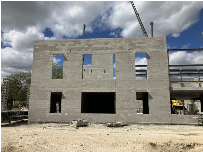
Masonry Wall – South Side of Area C
