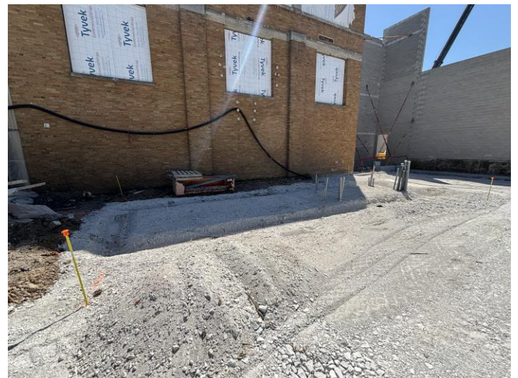
Generator Rough-In & Pad Staking
