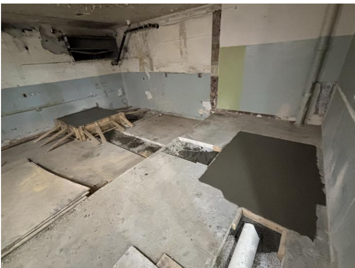
Column Pads – Area A
