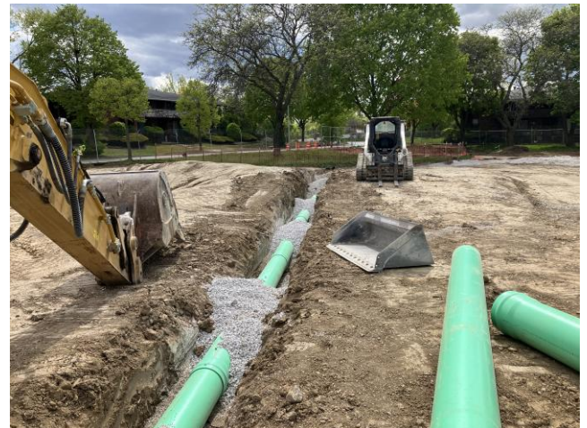
Site Underground Storm – South View
