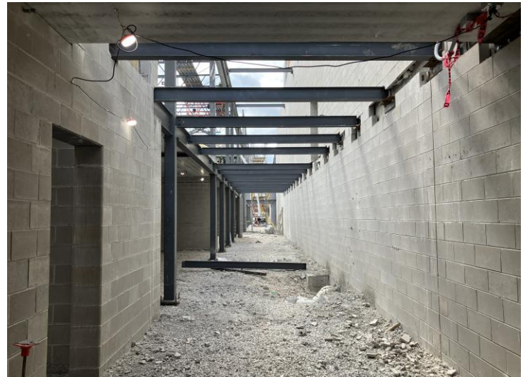
Structural Steel – East Side of Area B
