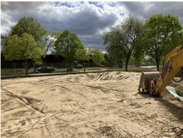
Pump Track – Southwest View
