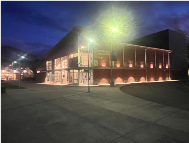
Existing lighting at main school entrance
