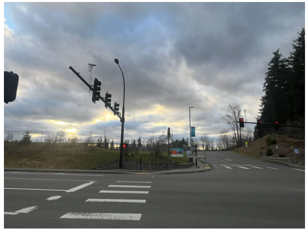
Looking north into site
