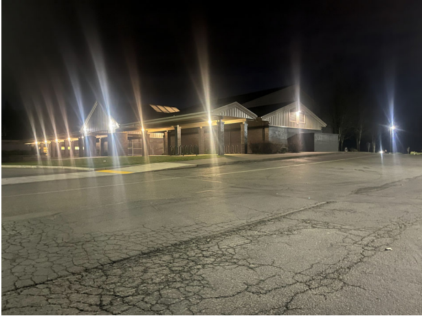
Existing lighting Mountain View Middle School
