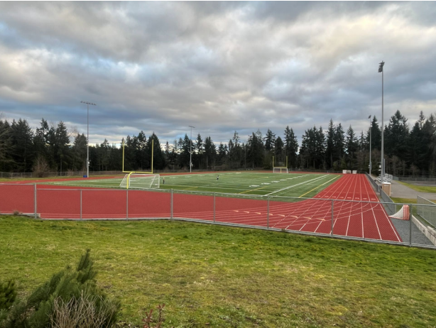
Existing football field lights Mountain View Middle School
