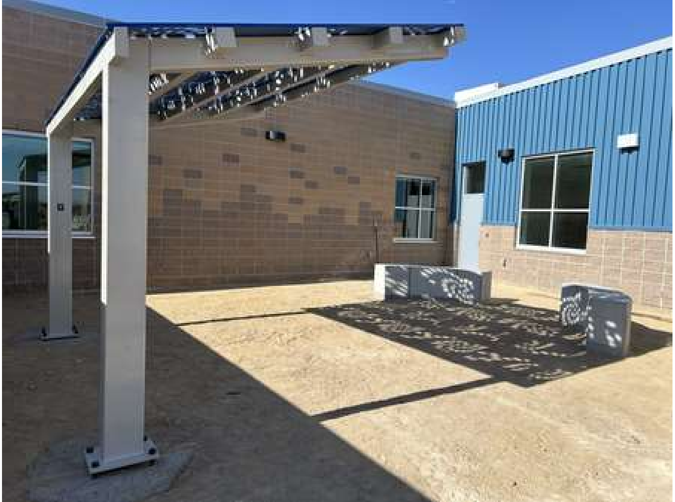
New Shade Structure
