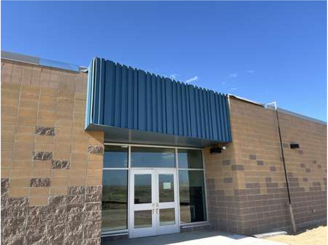
Sofit at Exterior Entrance
