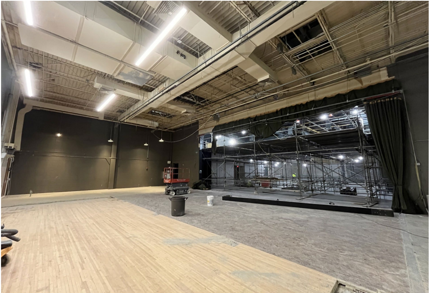
STAGE VIEW DEMOLITION
