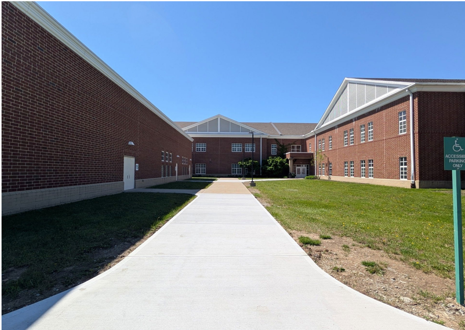
ZWMS SELECTIVE CONCRETE REPLACEMENT
