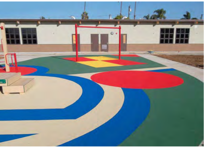
POURED-IN-PLACE SURFACING
