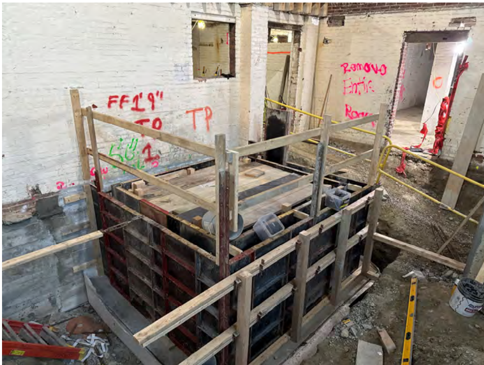
April 10: Elevator Shaft, Historic Building
