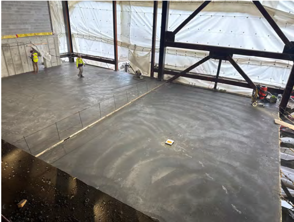
April 15: Multipurpose Room Slab-on-Grade
