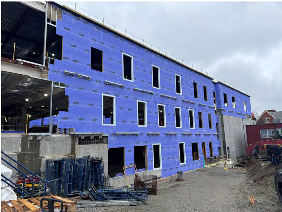
April 30: Exterior Sheathing Progress, East Elevation
