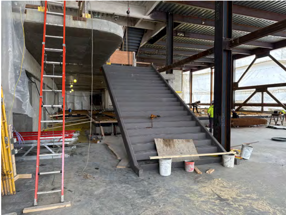
April 13: Installing Stair #3
