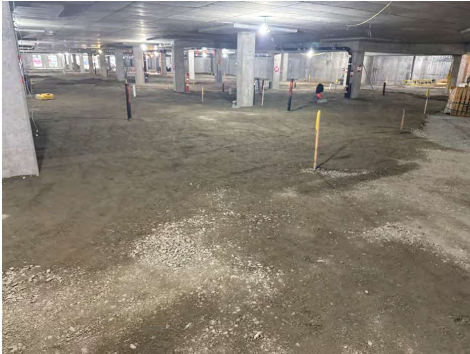
April 22: View of Garage Ready for Paving
