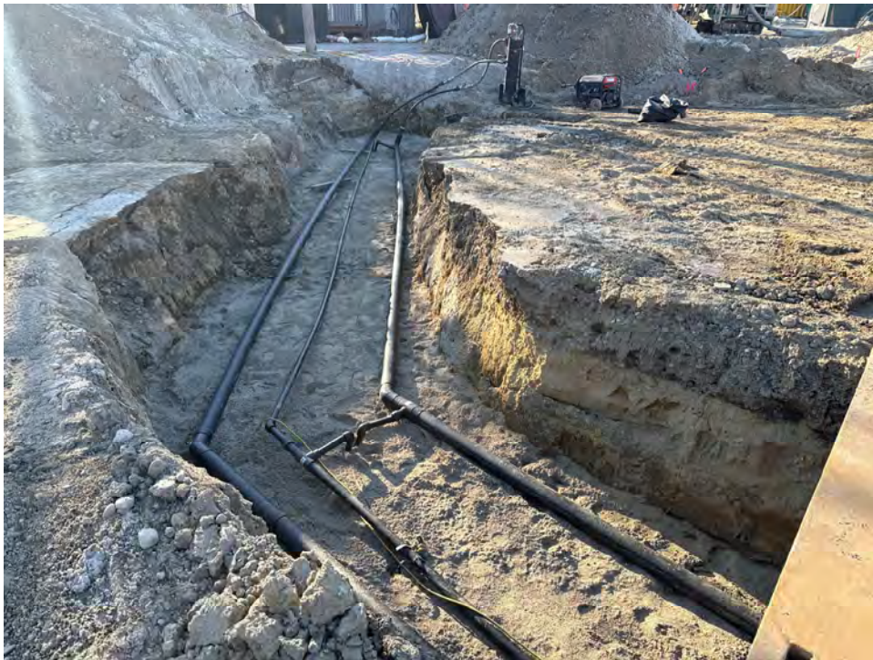
April 8: Geothermal Branch Installation
