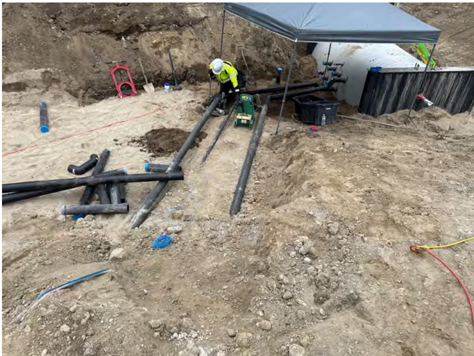
April 29: Geothermal Branches Tied Back to New Vault
