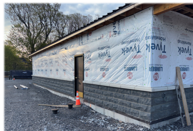
Concessions Ext. Masonry & In-wall MEP + Insulation
