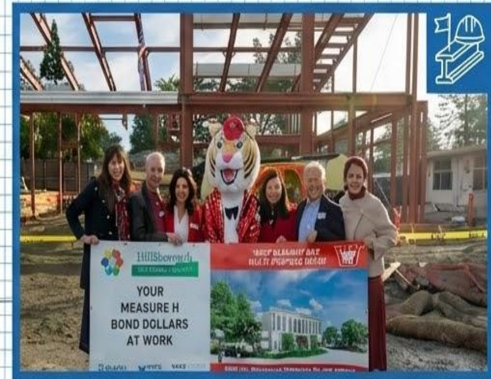
West "Topping Out" Event
