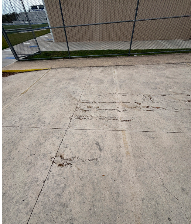
Deteriorating concrete
