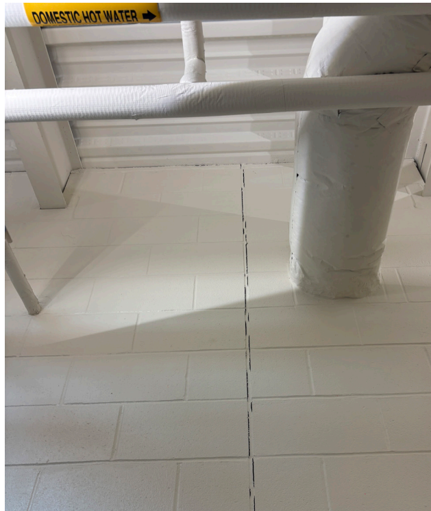
Deteriorating sealant
