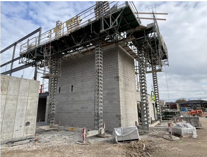
Stair Shaft Progress- Area C1
