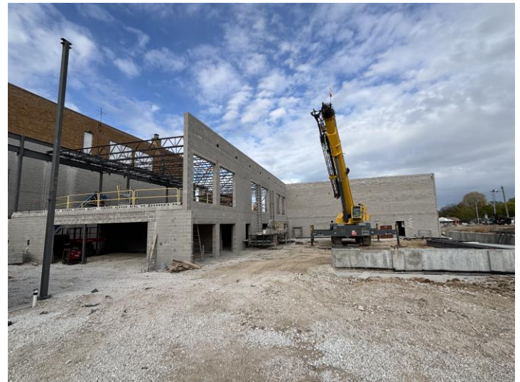
Steel Erection – View From Main Entry Through Natatorium
