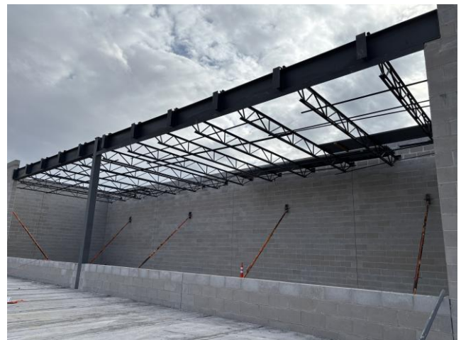
Steel Joist Installation– Area B1 Mechanical Room
