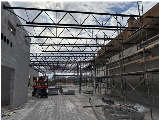
Steel Joist Installation- Area B1 Fitness & Weight Studio
