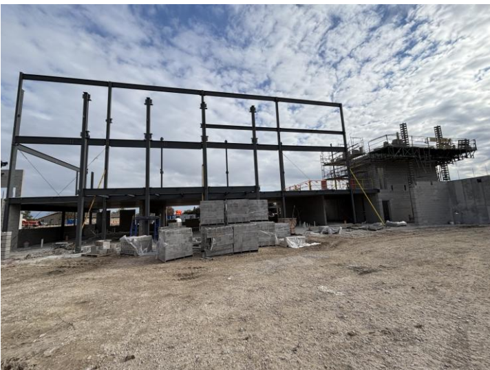
Steel Erection & CMU Stairwell Progress – Area C1
