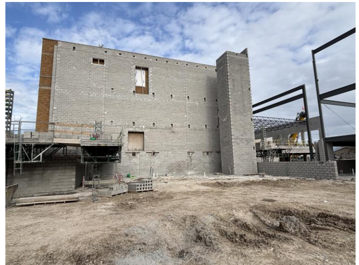
Elevator Shaft Top Out & Stair Shaft Progress- Area A2
