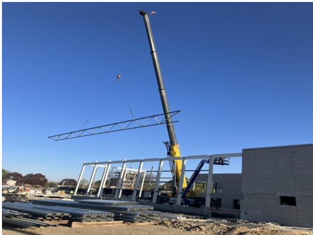
Structural Steel – South Side of Area C
