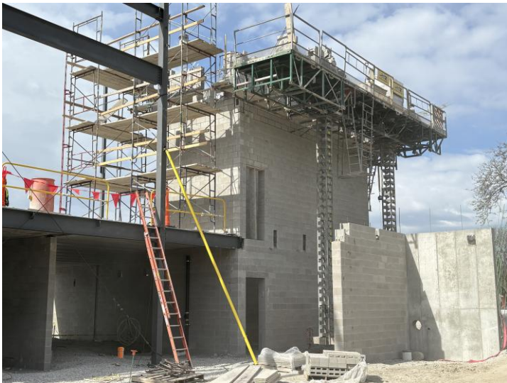
Masonry Staircase – West Side Area C
