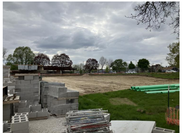
Site Grading – East Side of Tennis Courts
