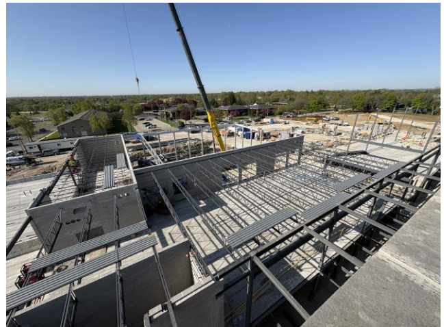
Joist Installation – Aerial View of Area B and C
