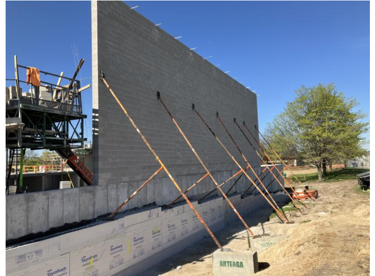
Masonry Wall – North Side of Area C
